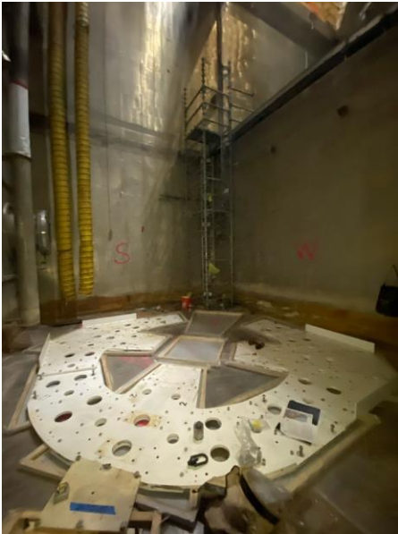
FTC Floor Plates Installed
