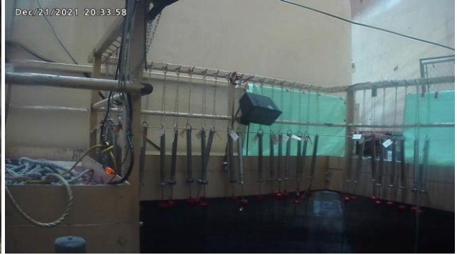
ICI pit with all ICI retracted and tethered in preparation for flood up and underwater segmentation
