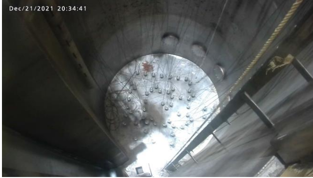
ICI pit with all ICI retracted and tethered in preparation for flood up and underwater segmentation
