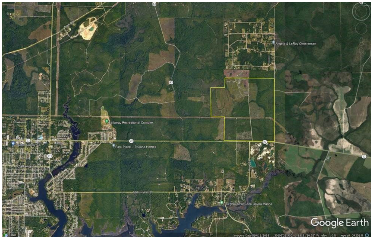
FIGURE 4.5 Bay Ranch Solar Project
