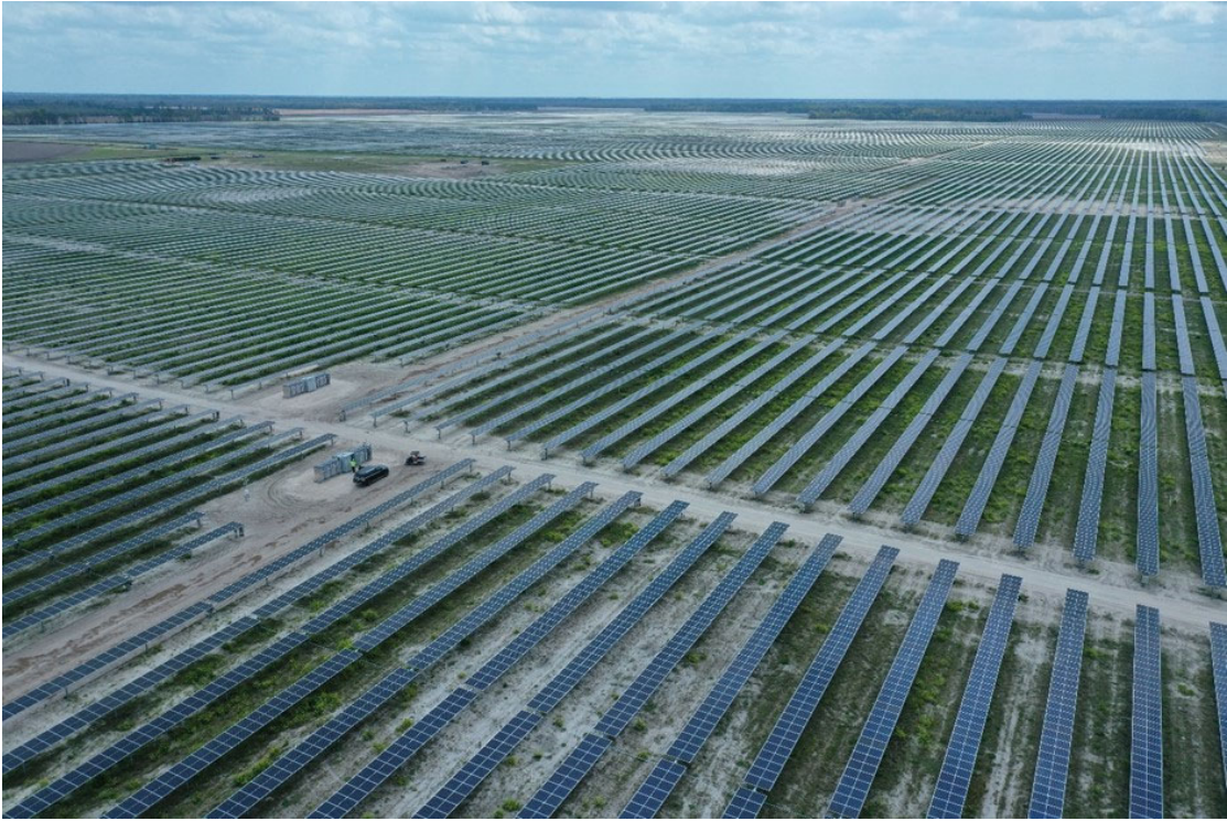
FIGURE 3.3 Twin Rivers Solar Power Plant
