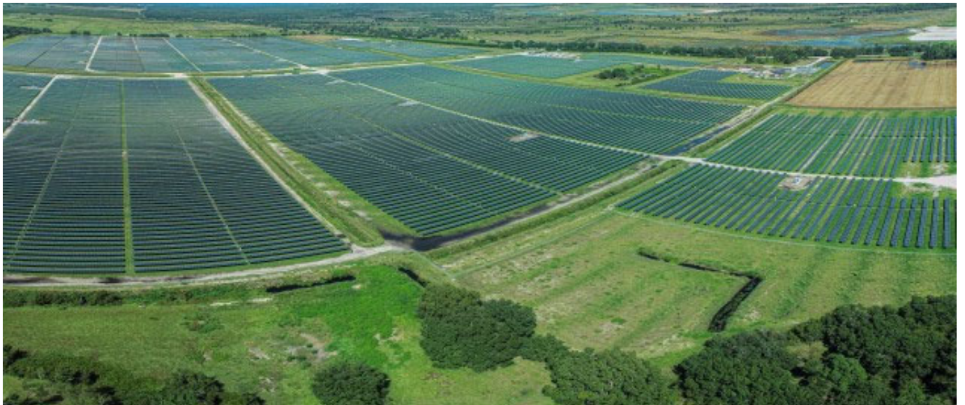
FIGURE 3.4 Duette Solar Power Plant
