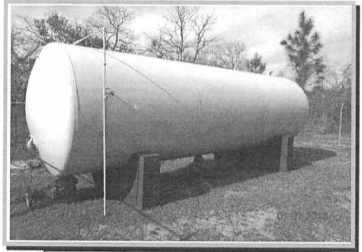
10,000 Gallon Ground Storage Tank at Plant #5
