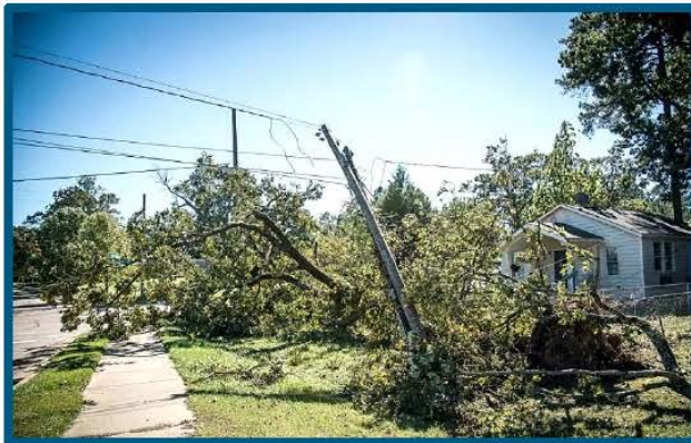
Figure 1: An example of residential customers that would be candidates for Undergrounding due to section of line and service in heavily vegetated areas.
