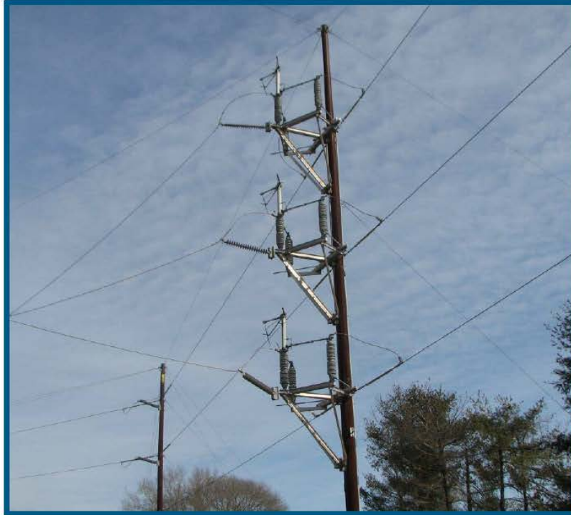
Figure 3: DEF Manually Operated Switch
