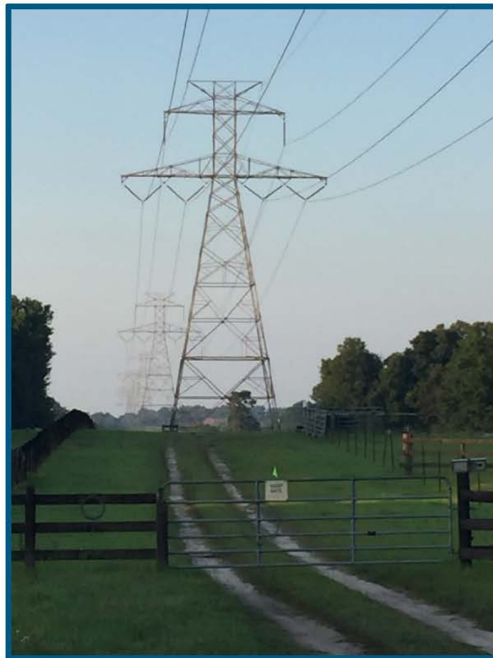
Figure 2: Double Circuit Tower
