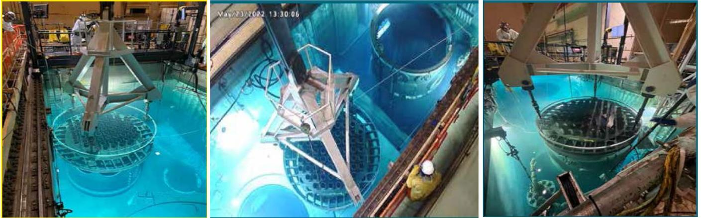
**Cutting Grout Holes in Plenum**
