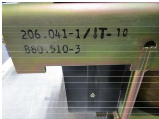
As Received Left Side of Breaker Platform
