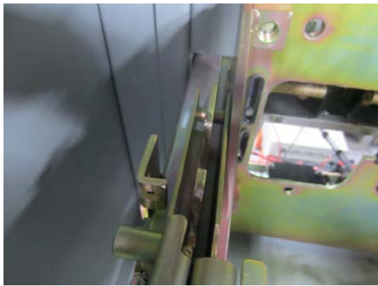
Breaker Frame Located in the Connect Position Stop Bracket
