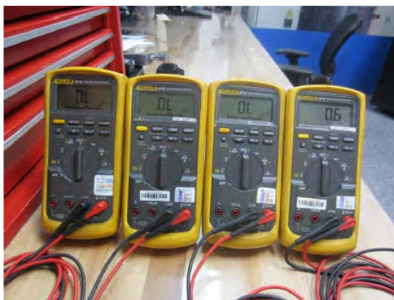
Breaker Closed Switch Position
