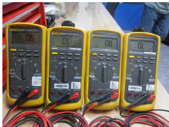
Breaker Open Switch Position
