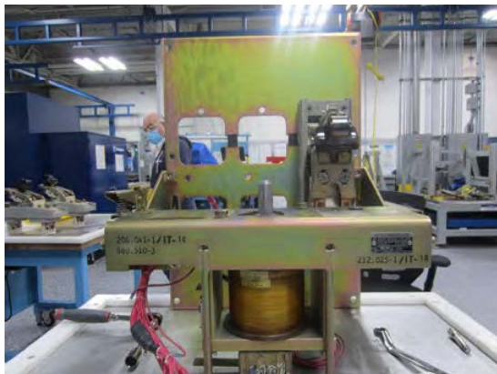
Phase 'B' Removed
