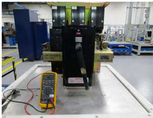
Breaker Closed, Switch Contact Open
