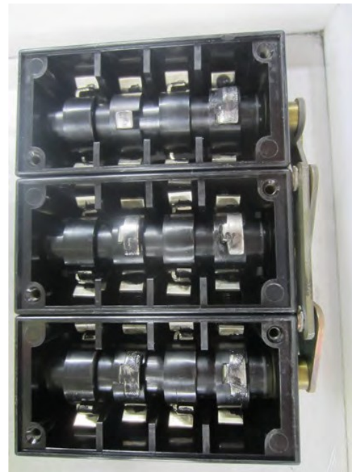
Rear of Auxiliary Switches
