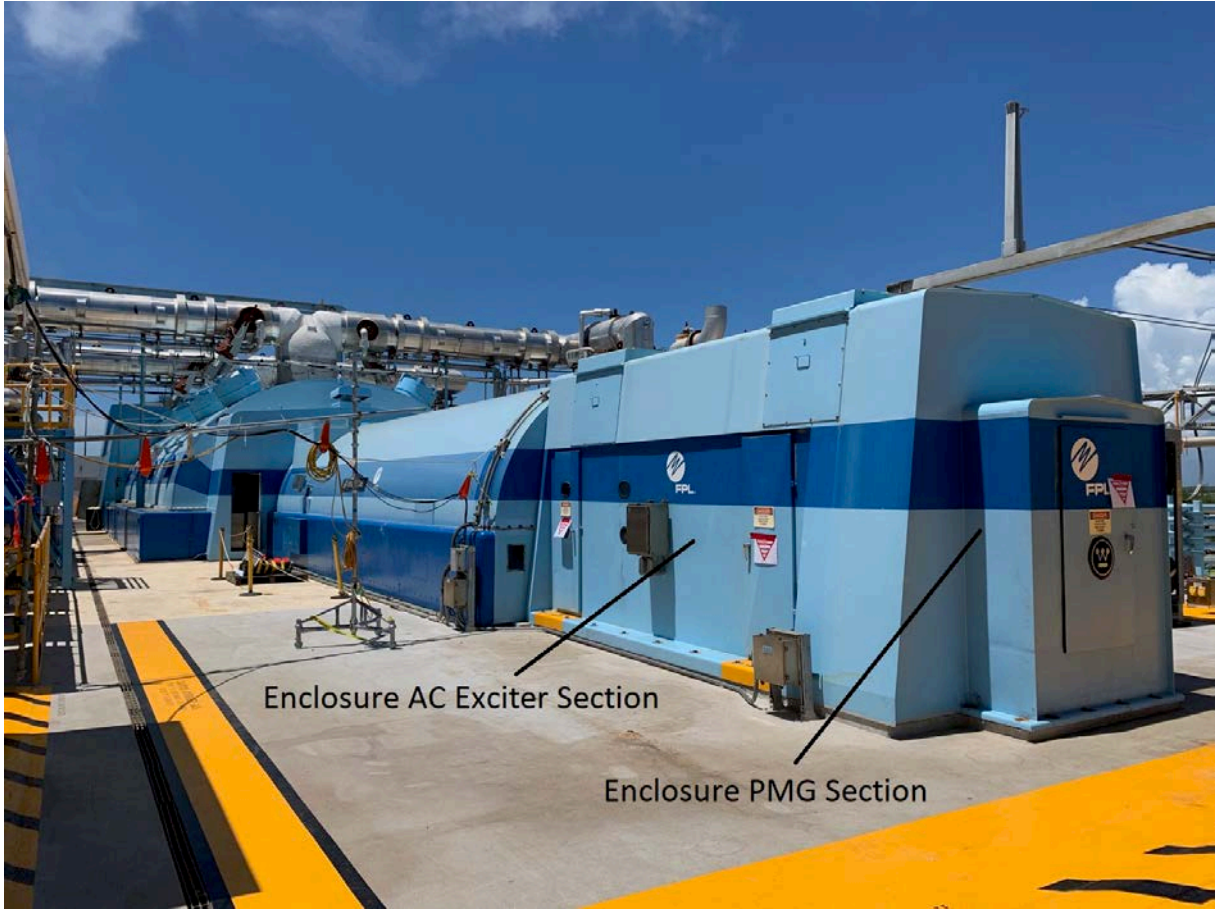
Fig. 1 U4 Exciter Housing
