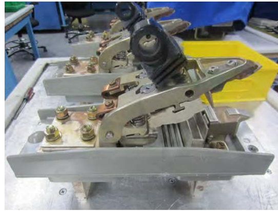
Phase 'C' Removed
