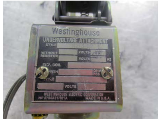
UVTA Assembly Removed
