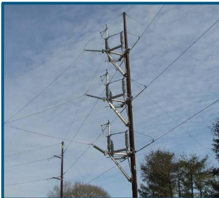
Figure 3: DEF Manually Operated Switch
