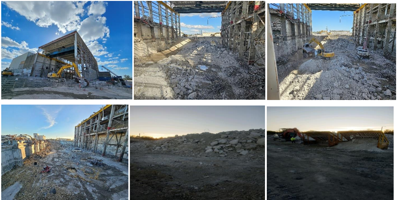
Plant Admin Building Demolition
