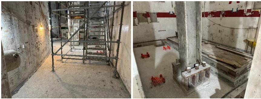
Turbine Building Demolition
