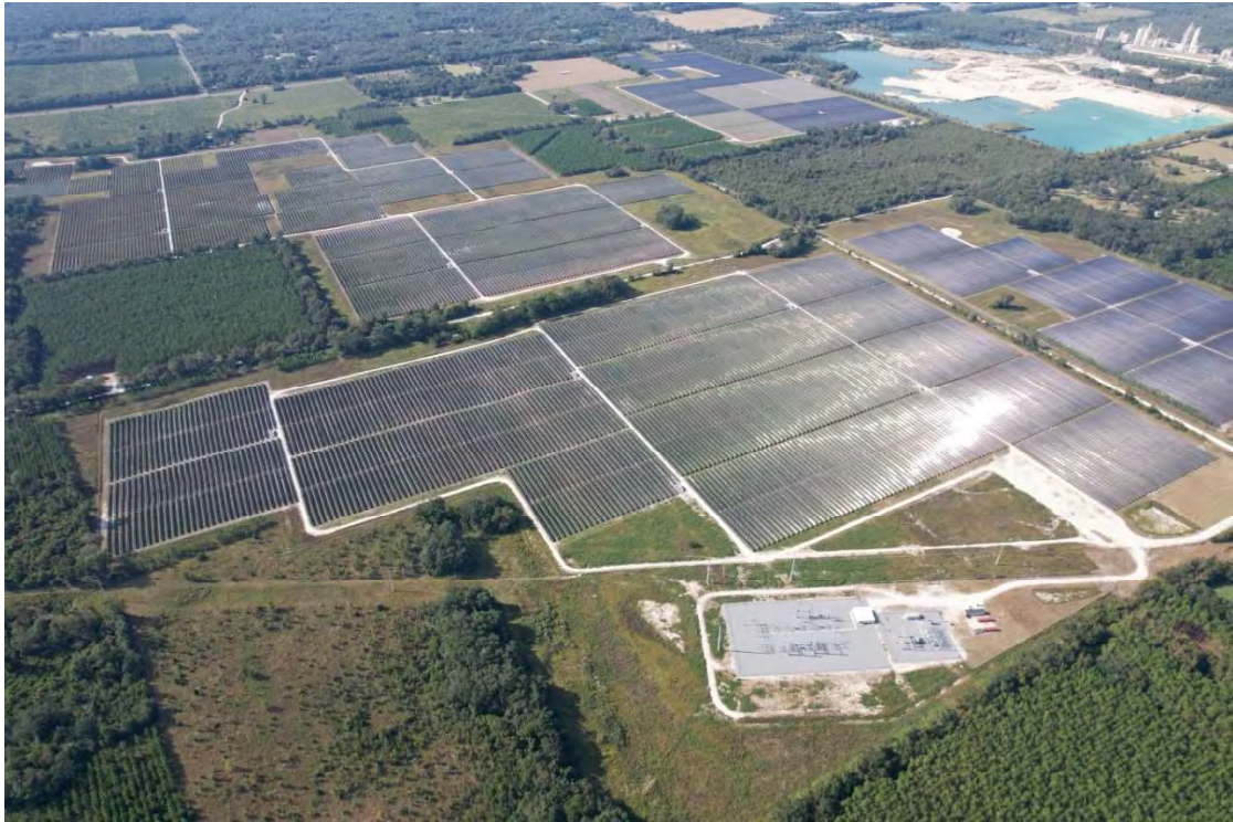
FIGURE 3.5 Hildreth Power Plant
