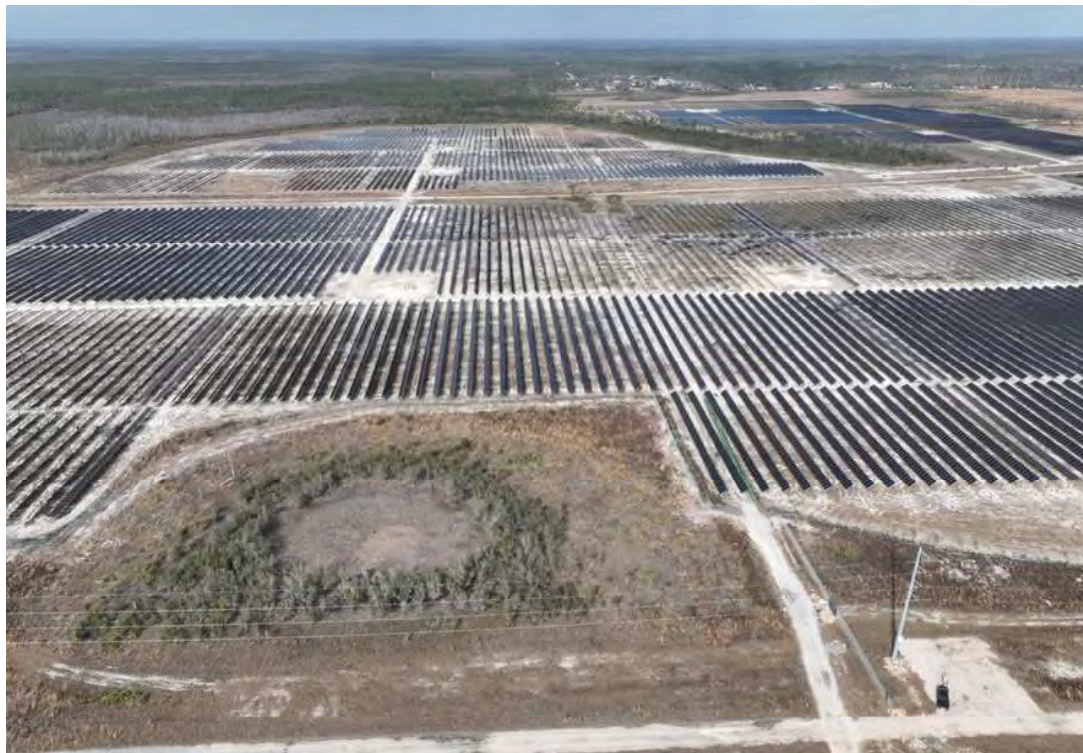
FIGURE 3.2 Bay Ranch Solar Power Plant
