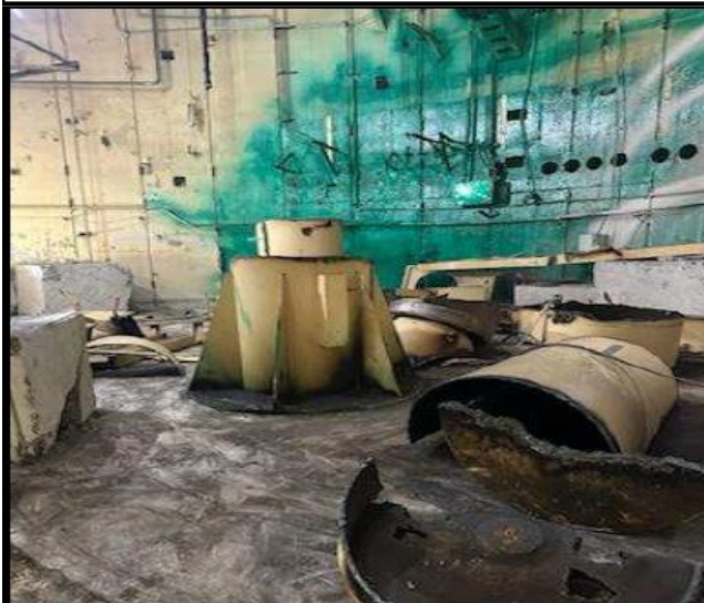
RB 119' Components Removal
