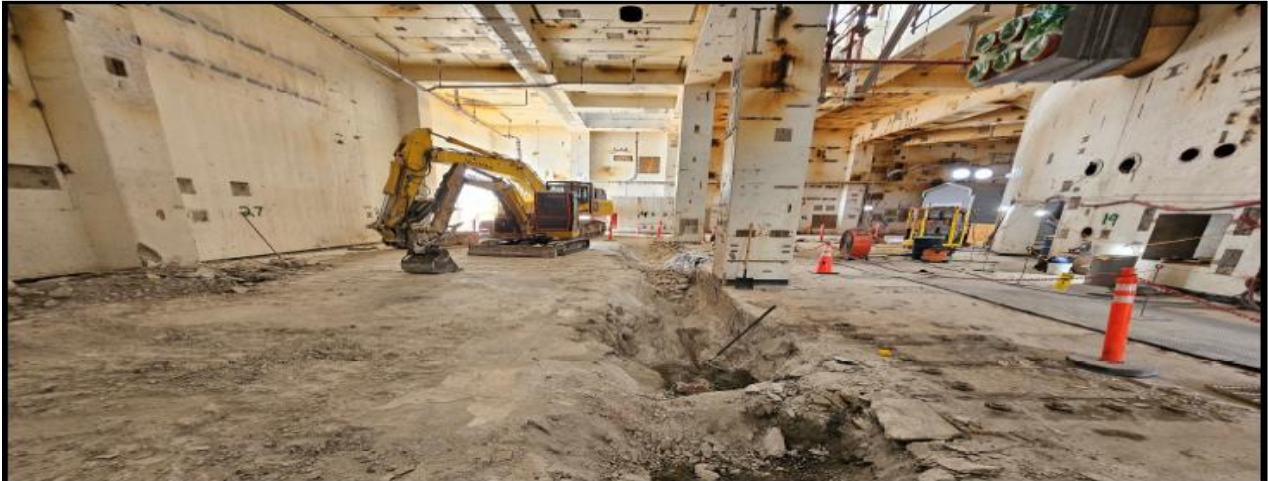
IB 119 Drains Removal
