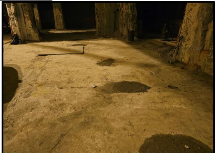
AB 119' Filling Drains with Concrete
