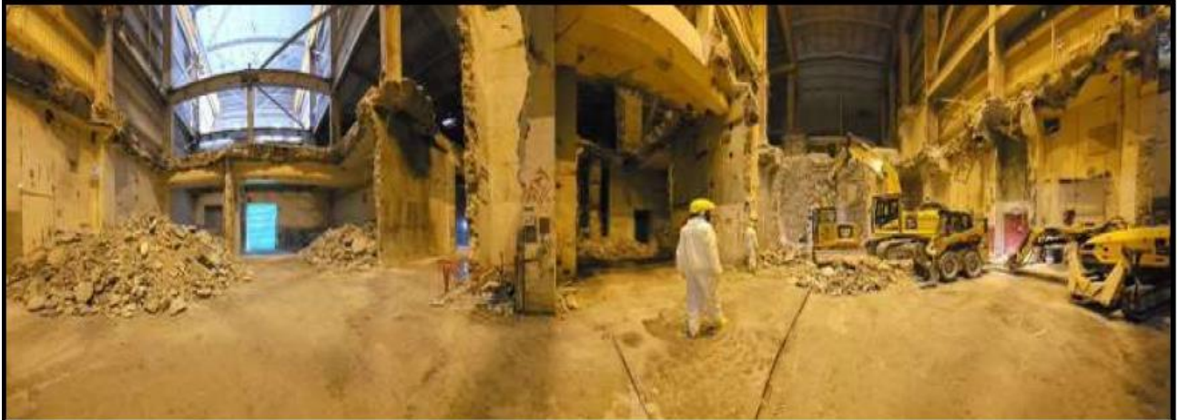
AB 119' Phase 3 Demolition
