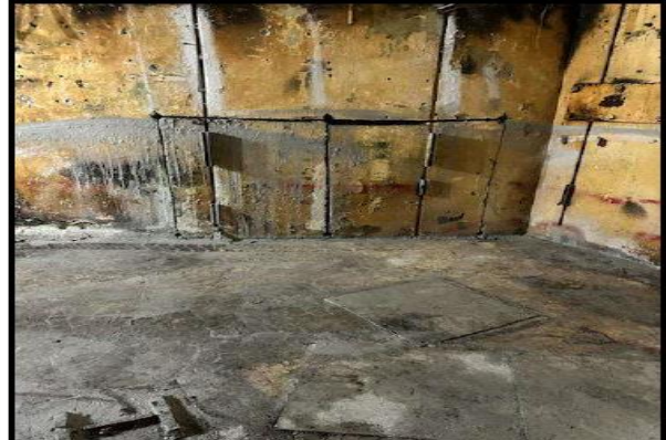
RB 119' Wall Openings
