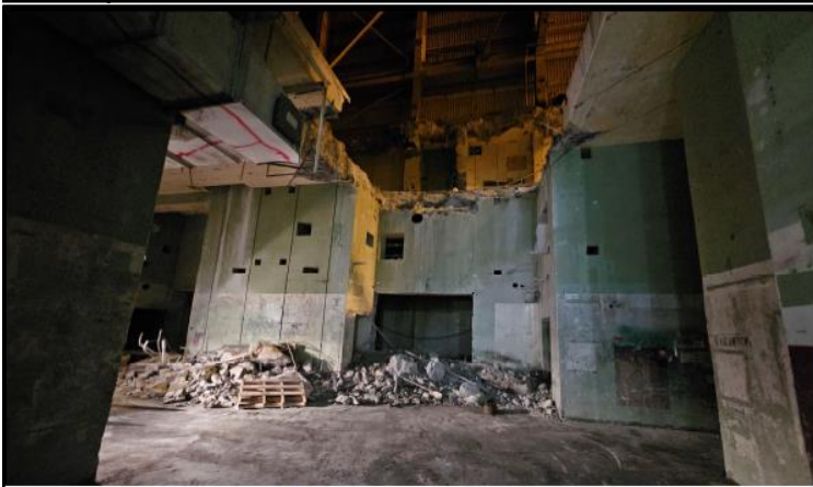
AB 95' Phase 3 Demolition
