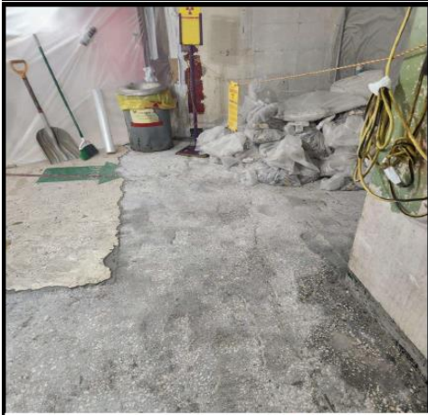
IB 119 Decon Coating Removal
