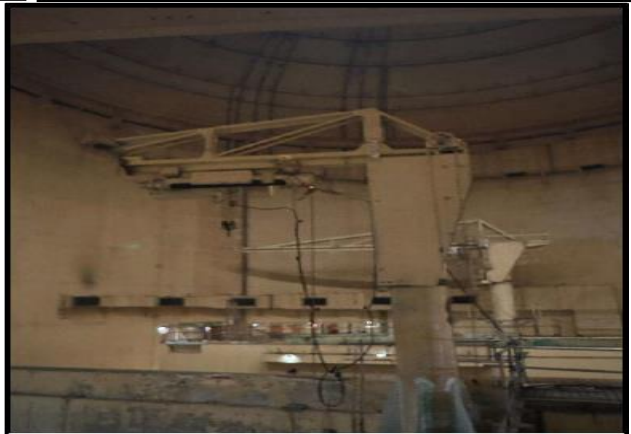
RB 119' Components Removal
