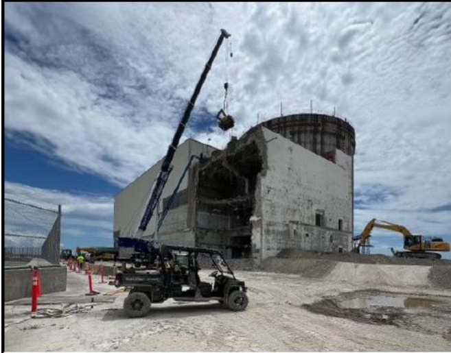
Raised Brokk to Control Complex Roof
