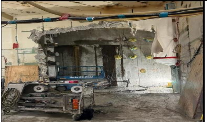
RB South Wall Opening
