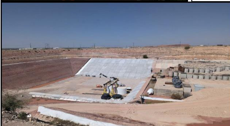
CR3 Top Package Final Resting Place
