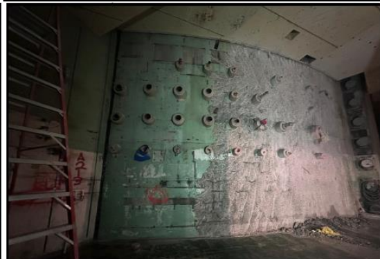
AB 119' Decon Paint Coating Removal RB Wall
