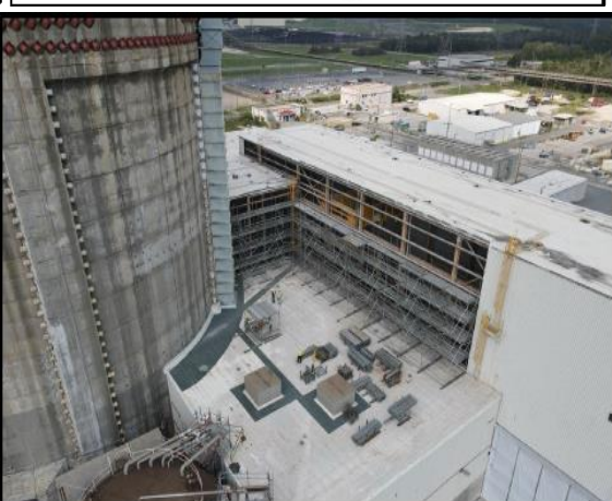
AB Galbestos Siding Removal
