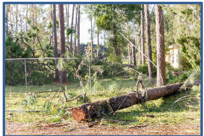
Figure 2: Section of lines that runs through backlot and heavily vegetated areas that is a candidate for Undergrounding.
