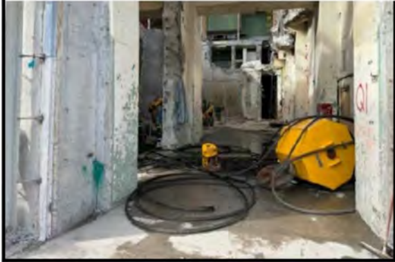
AB Super Structure -Cutting Crane Blocks and Cables
