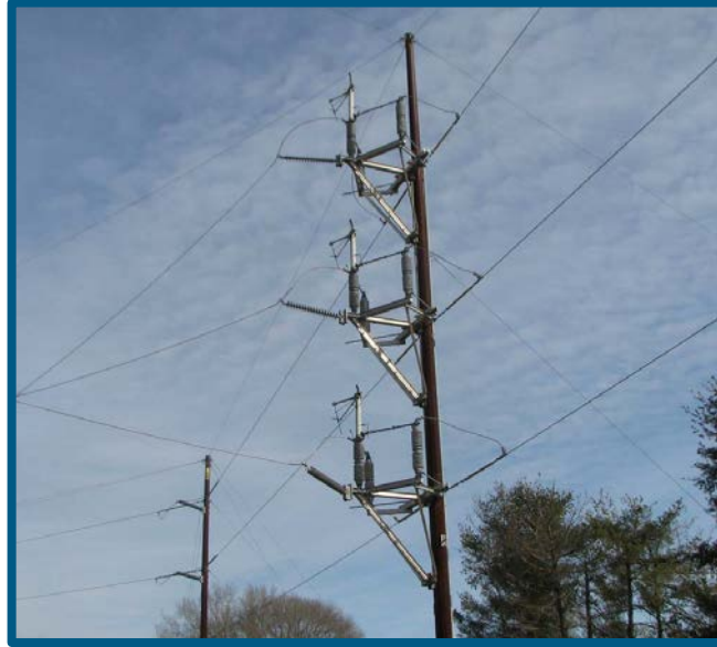
Figure 5: DEF Manually Operated Switch
