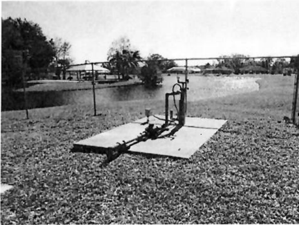
Photo 1: Overview of well.
