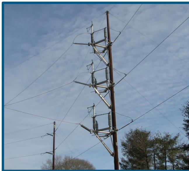
Figure 5: DEF Manually Operated Switch
