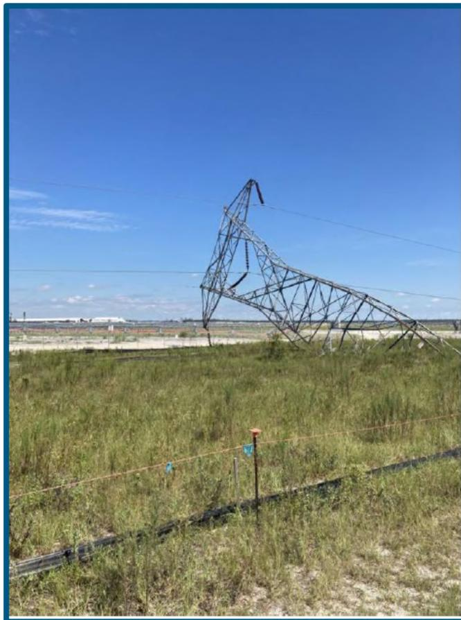
Figure 4: Lattice Tower impacted by Hurricane Idalia
