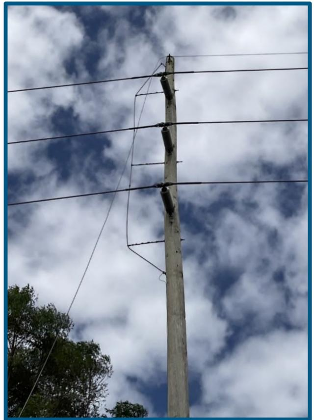
*Figure 2: Broken Static due to extreme weather event.*
