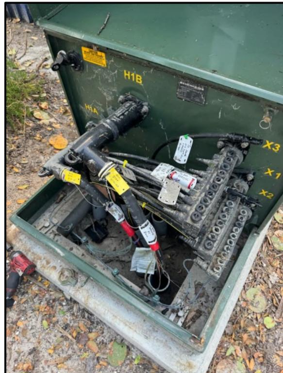
Figure 2: Underground construction with sealed connectors mitigating impacts of storm surge.
