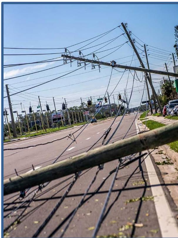
*Figure 1: Distribution feeder poles broken by straight line winds from Category 3 hurricane.*
