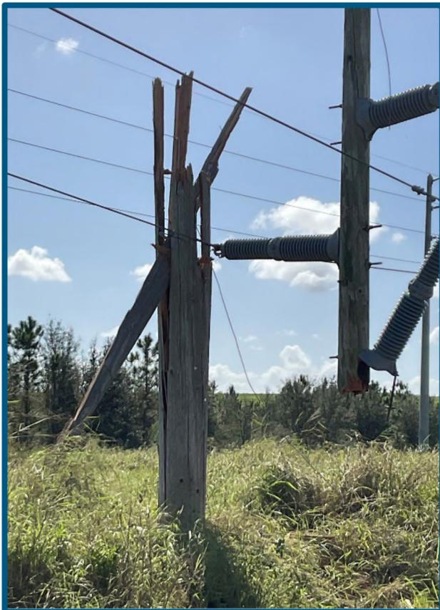
*Figure 1: Broken Pole due to extreme weather event.*
