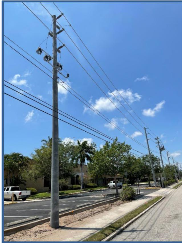
*Figure 2: Hardened distribution feeder including structures that have been strengthened to the NESC 250C standard and increased BIL from hardware and spacing upgrades.*
