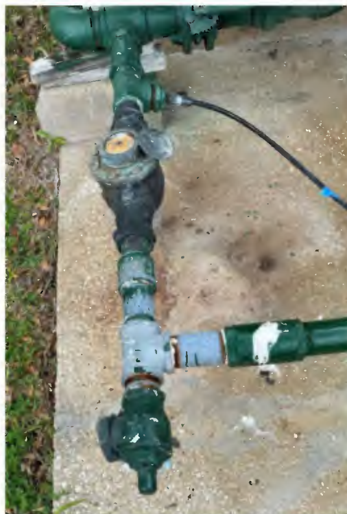
Figure 2-2: Well Meter
