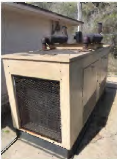
Figure 2-9: Back-up Power Generator
