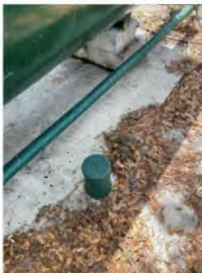
Figure 2-5: Collapsed Well
