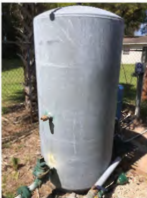
Figure 2-4: Patch on Storage Tank
