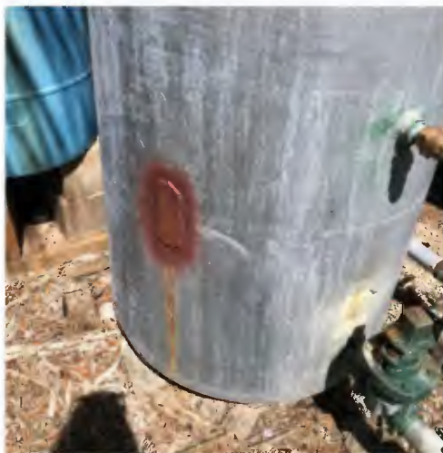
Figure 2-4: Patch on Storage Tank
