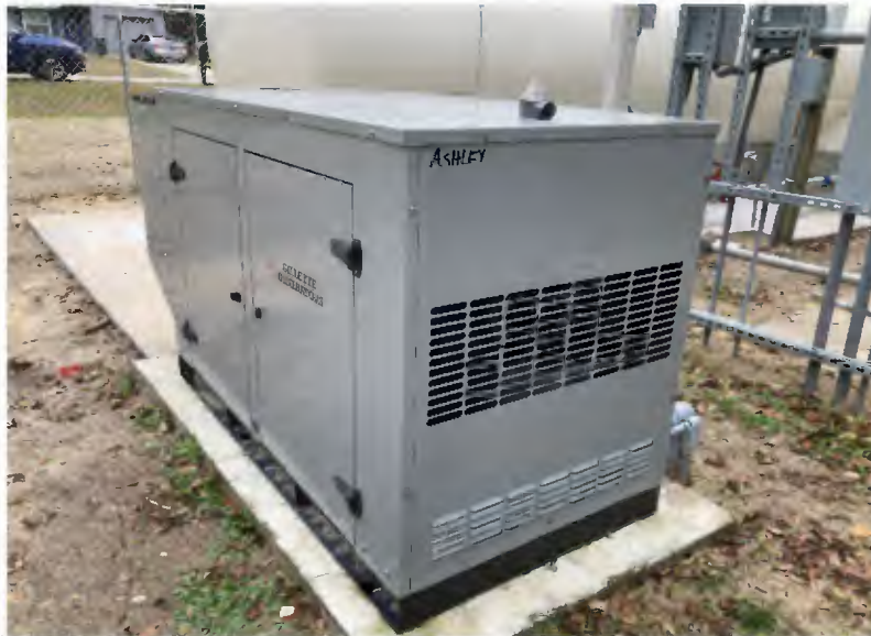
Emergency generator installation - Ashely Heights system.
