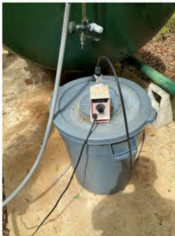
Figure 2-4: Chlorine Treatment Bin
