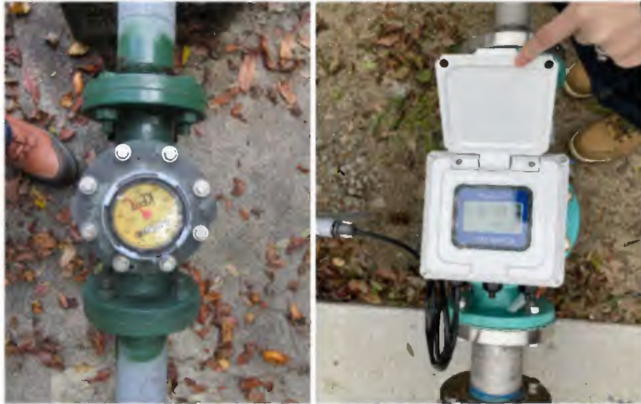
Before (Left) & After (Right): Flow Meter Replacement - Asheley Heights system
