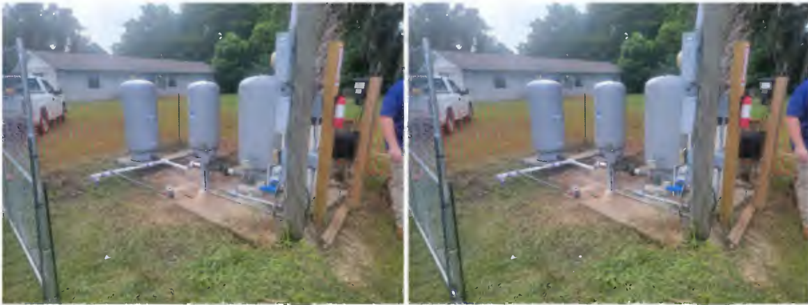
Temporary tanks installed after closing pending installation of a new hydropneumatic tank – Oakcrest Villas system
