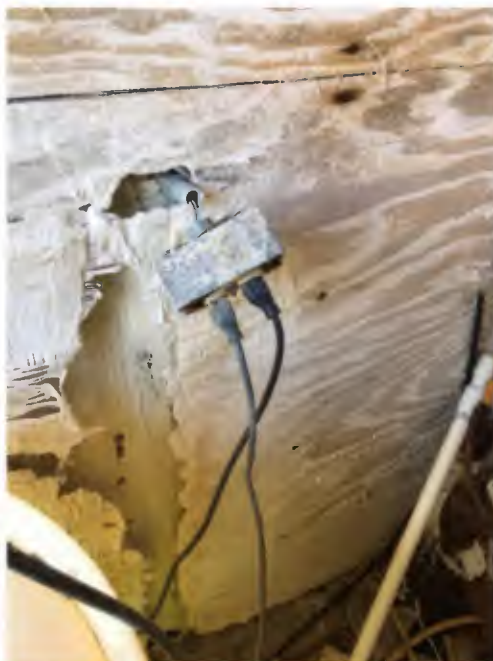
Figure 2-4: Chemical Pump Outlet
