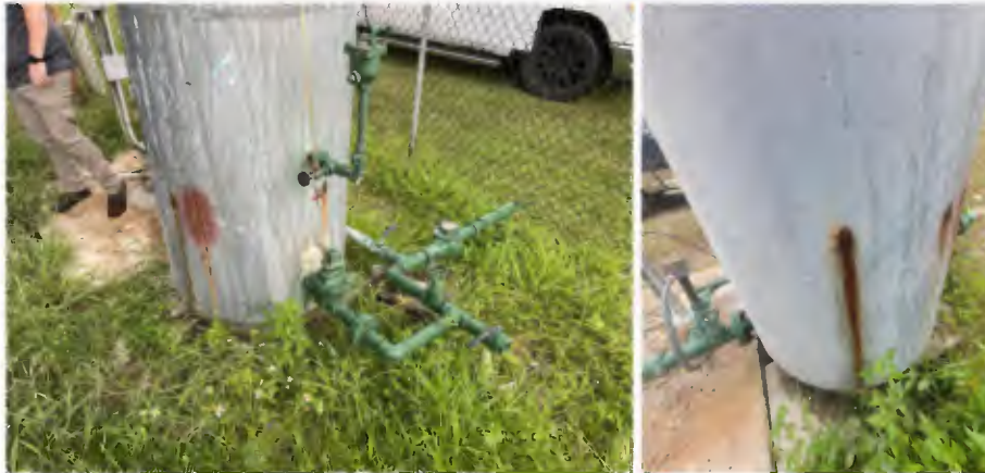
Rust and leaks appearing prior to hydrpneumatic tank failure – Oakcrest Villas system
