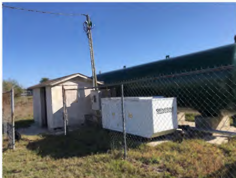
Figure 2-6: Generator and Pump Station Building
