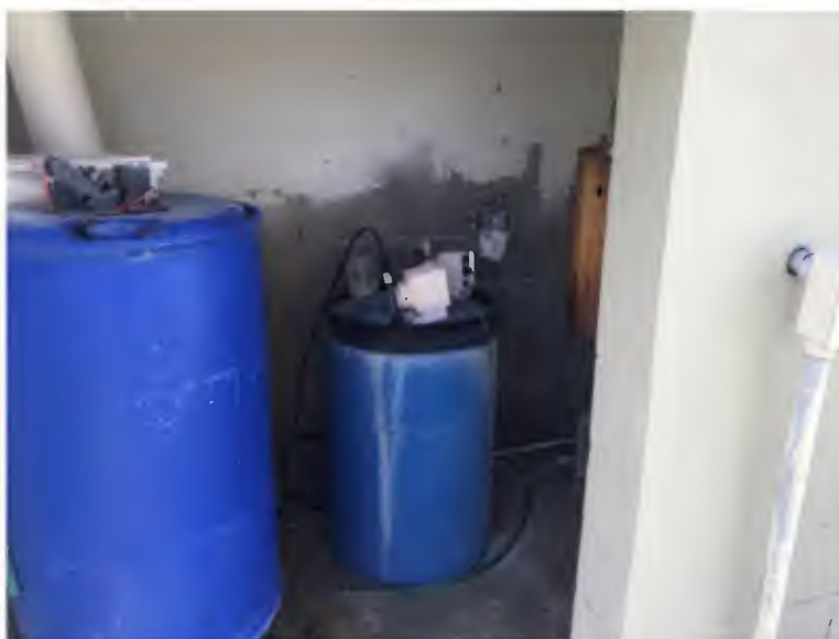
Figure 2-8: Chlorine Treatment
