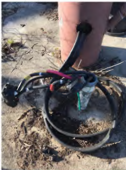
Figure 2-8: Exposed Conduit on Well 2
