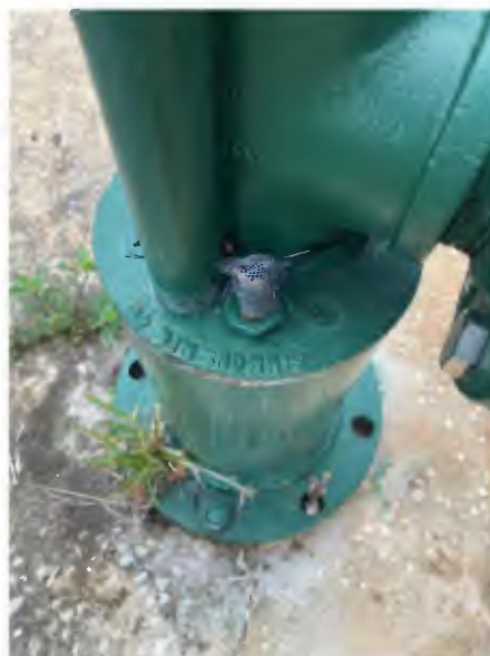
Figure 2-2: Well 1 3/4 -Inch Screened Vent
