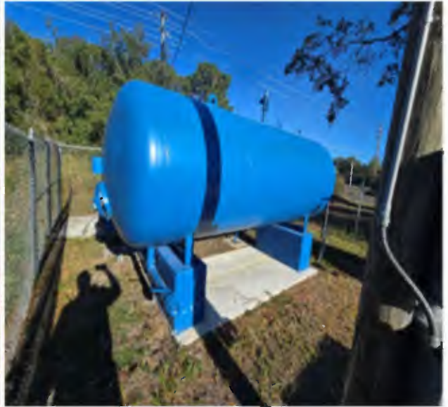
Before (Left) & After (Right): Hydropneumatic tank replacement - Belleview Oaks Estates system.
