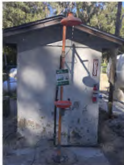
Emergency eye wash station - Ashely Heights system (Note: Similar installations at other systems, as requirea).
