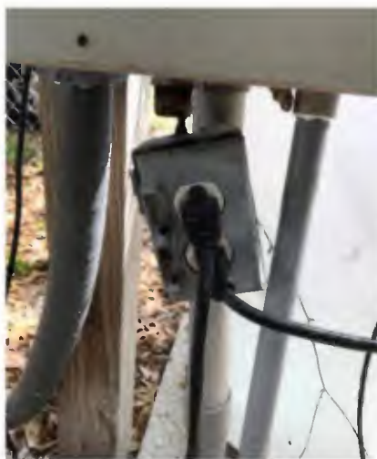
Figure 2-5: Well Starter Outlet
