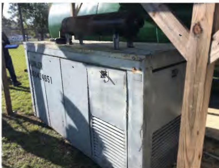
Figure 2-6: Back-up Power Generator
