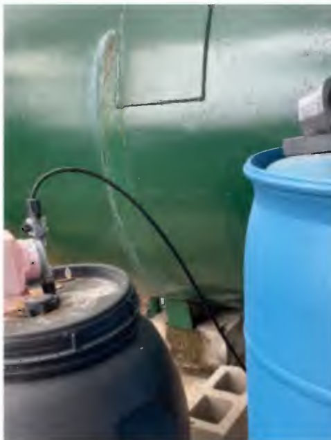
Figure 2-8: Rust on Storage Tank
