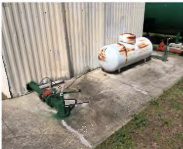
Figure 2-2: Combined Source Meter
