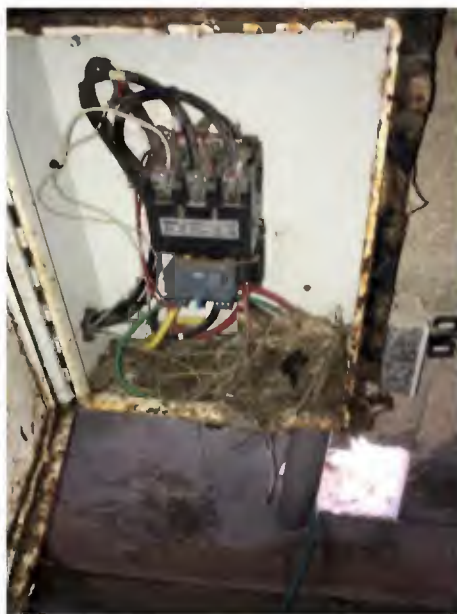
Figure 2-10: Debris Build-Up in Panel
