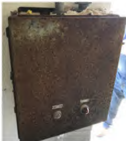
Figure 2-12: Rusted Electrical Panel
