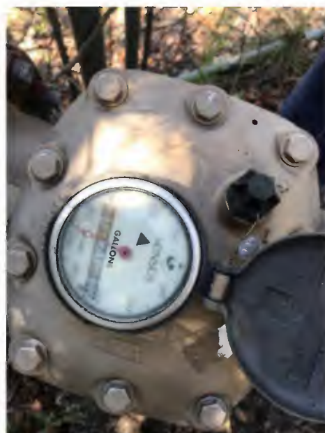
Figure 2-5: Well 2 Flow Meter
