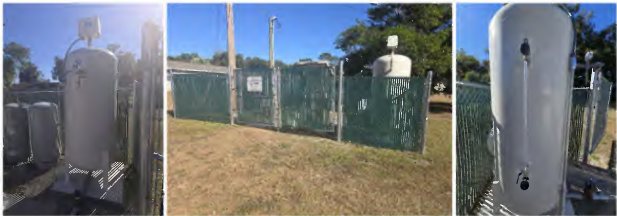
New hydropneumatics tank and fencing – Oakcrest Villas system
