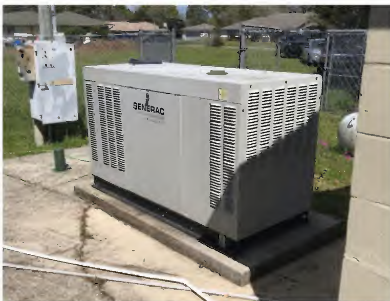
Figure 2-11: Back-up Power Generator
