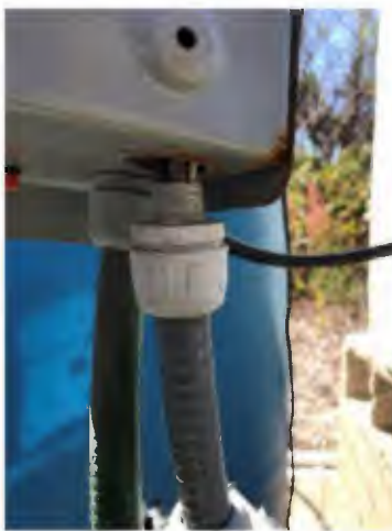
Figure 2-9: WTP 1 Well Pump Exposed Wires
