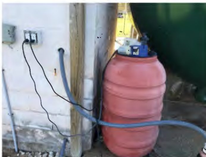
Figure 2-4: Chlorine Treatment
