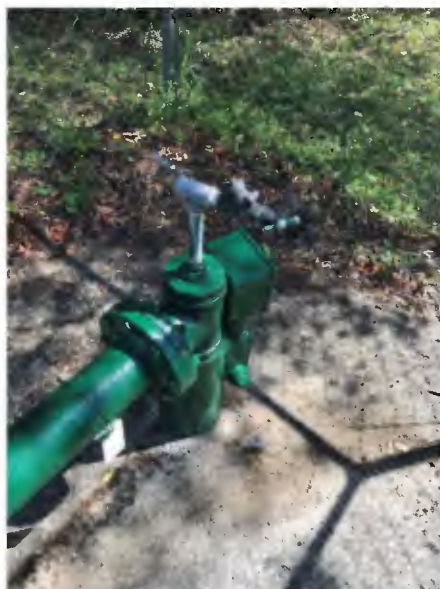
Figure 2-5: Well 3 Meter
