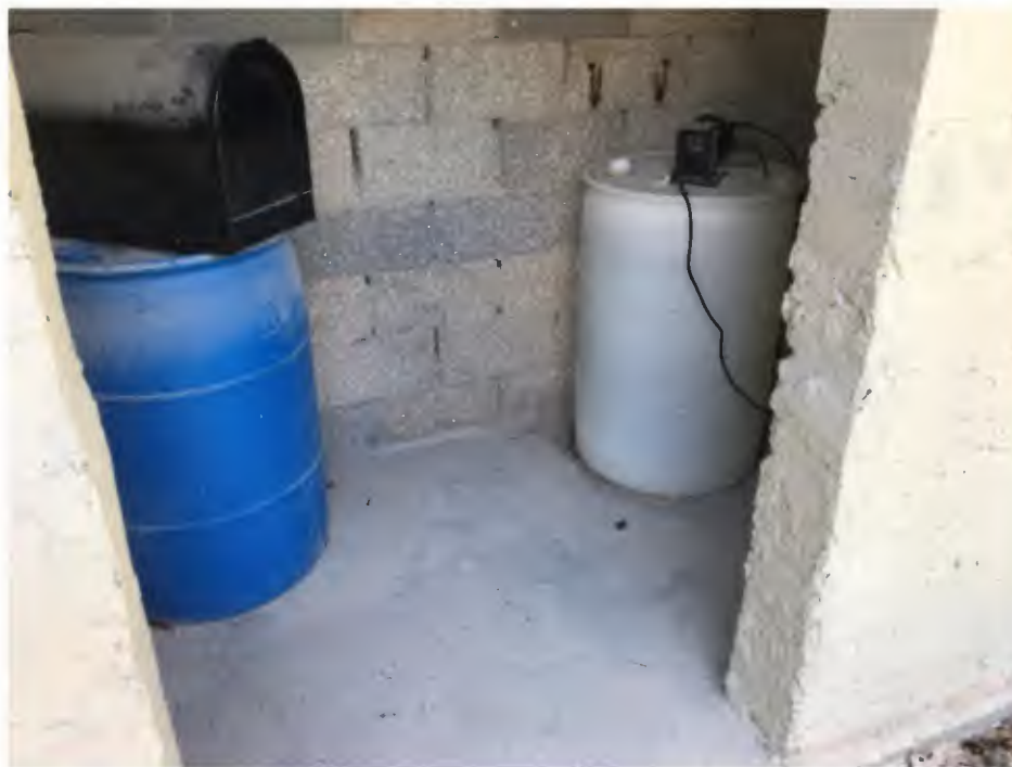
Figure 2-2: Chlorine Treatment
