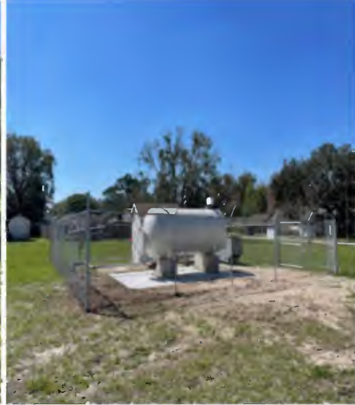
Before (Left) & After (Right): Hydropneumatic tank replacement - Ponderosa Pines system.
