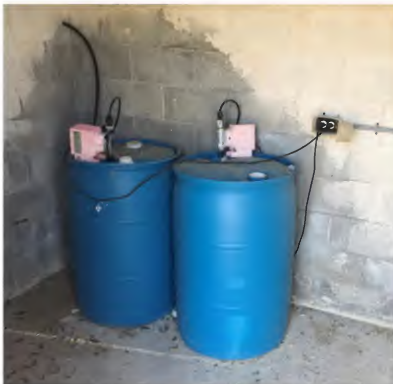
Figure 2-3: Chemical Treatment
