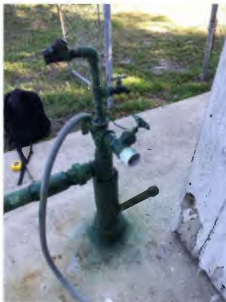
Figure 2-4: Terrace Well Source Meter
