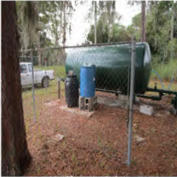
Before (Left) & After (Right): Hydropneumatic tank replacement - Belleview Oaks Estates system.
