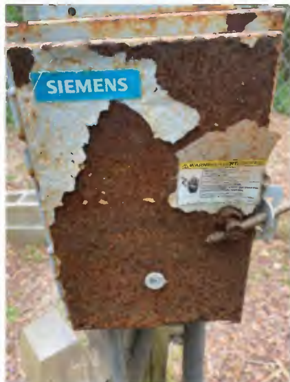
Figure 2-6: Corroded Pump Starter Box
