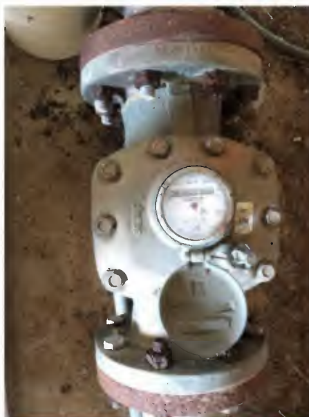
Figure 2-2: Combined Source Meter
