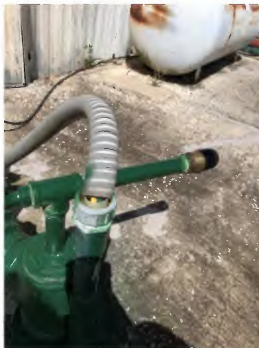
Figure 2-9: Exposed Conduit Wires on Well 2
