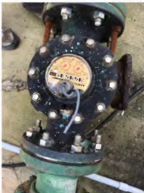
Figure 2-3: Well 1 Flow Meter
