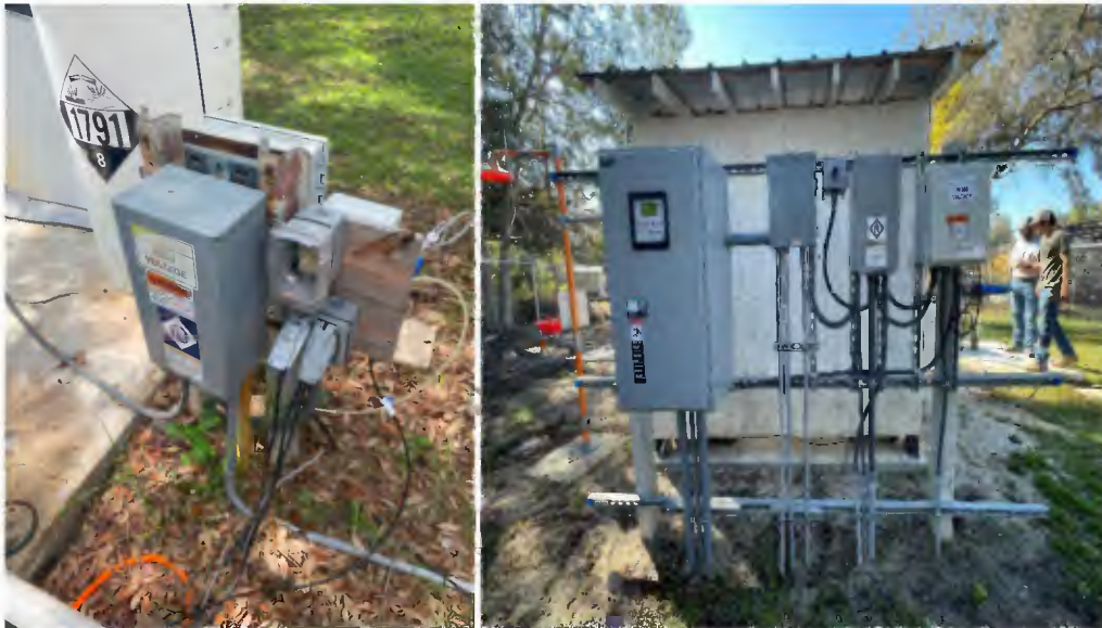
Before (Left) & After (Right): Electrical panel improvements - Ponderosa Pines system.
