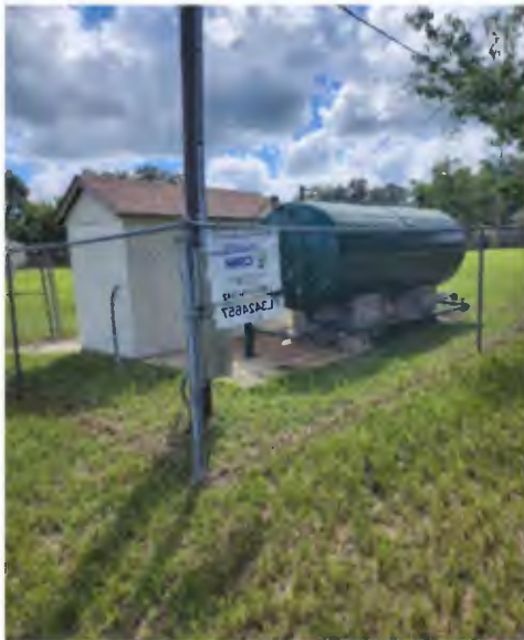
Before (Left) & After (Right): Hydropneumatic tank replacement - Country Walk system.
