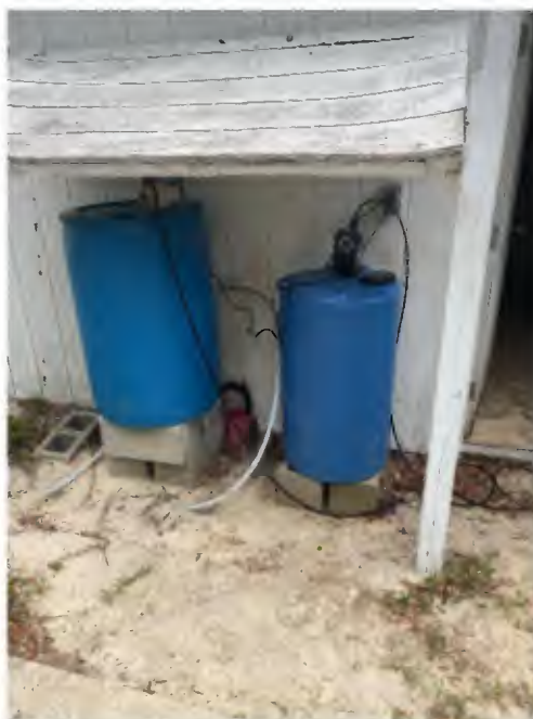
Figure 2-4: Chlorine Treatment
