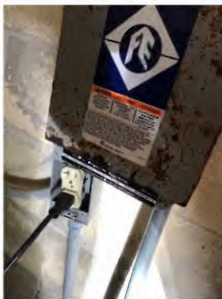
Figure 2-6: Rusty Pump Starter Panel
