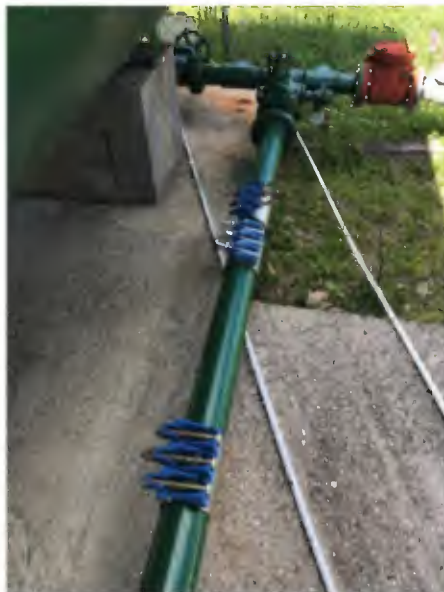
Figure 2-9: Leak Repairs on Bypass Piping
