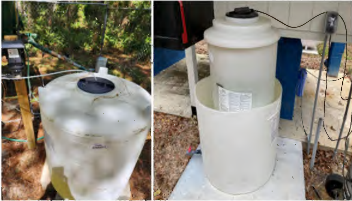
Before (Left) & After (Right): Chemical containment and shade structure - Emil-Mar system.
