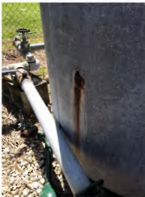
Figure 2-5: Storage Tank Leak
