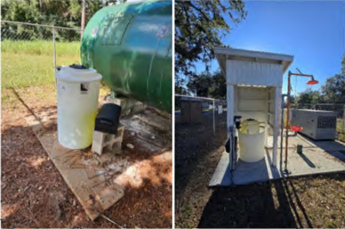
Before (Left) & After (Right): Disinfection system improvements (shade structure and containment) - Bellevue Oaks Estates system.
