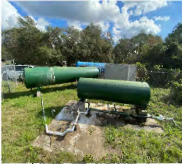
Before (Left) & After (Right): Hydropneumatic tank replacement - Ponderosa Pines system.
