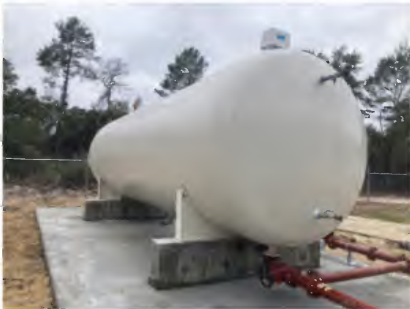
Before (Left) & After (Right): Hydropneumatic tank replacement - Winding Waters system.
