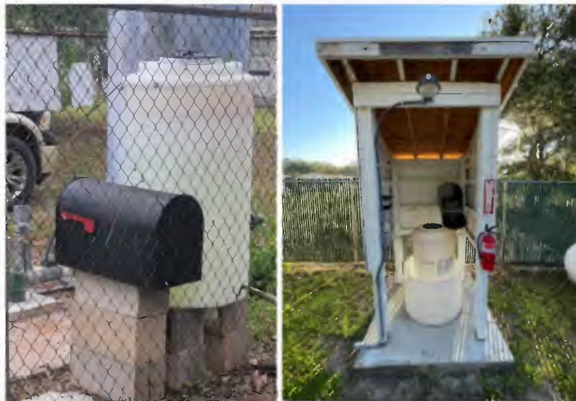
Before (Left) & After (Right): New Chemical containment and shade structure - Oakcrest Villas system.
