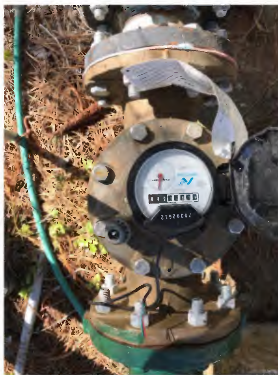
Figure 2-6: Distribution Meter
