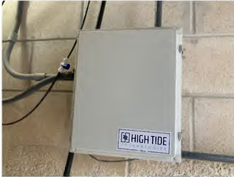
Remote monitoring unit - Florida Heights system (Note: The same equipment has been installed at all 23 Sunshine systems).
