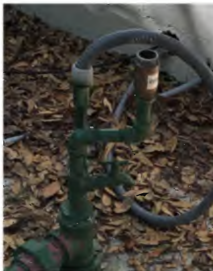
Figure 2-7: Unscreened Well Vent
