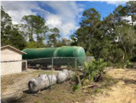
Before (Left) & After (Right): Hydropneumatic tank replacement - Winding Waters system.
