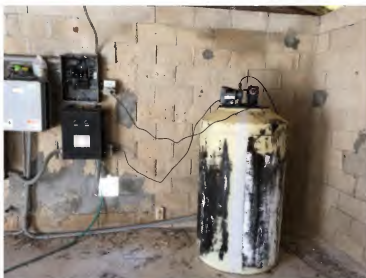
Figure 2-4: Chlorine Treatment
