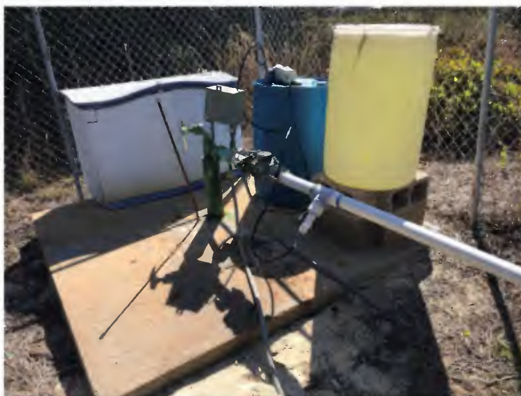
Figure 2-3: WTP 1 Chlorine Treatment
