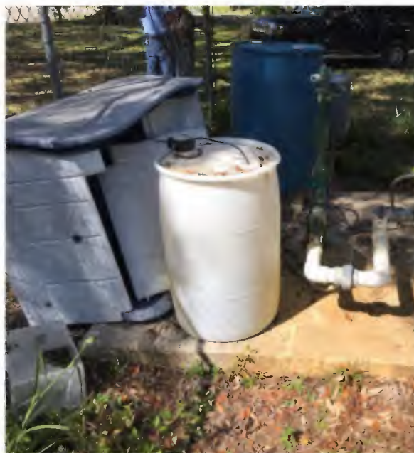
Figure 2-4: WTP 2 Chlorine Treatment
