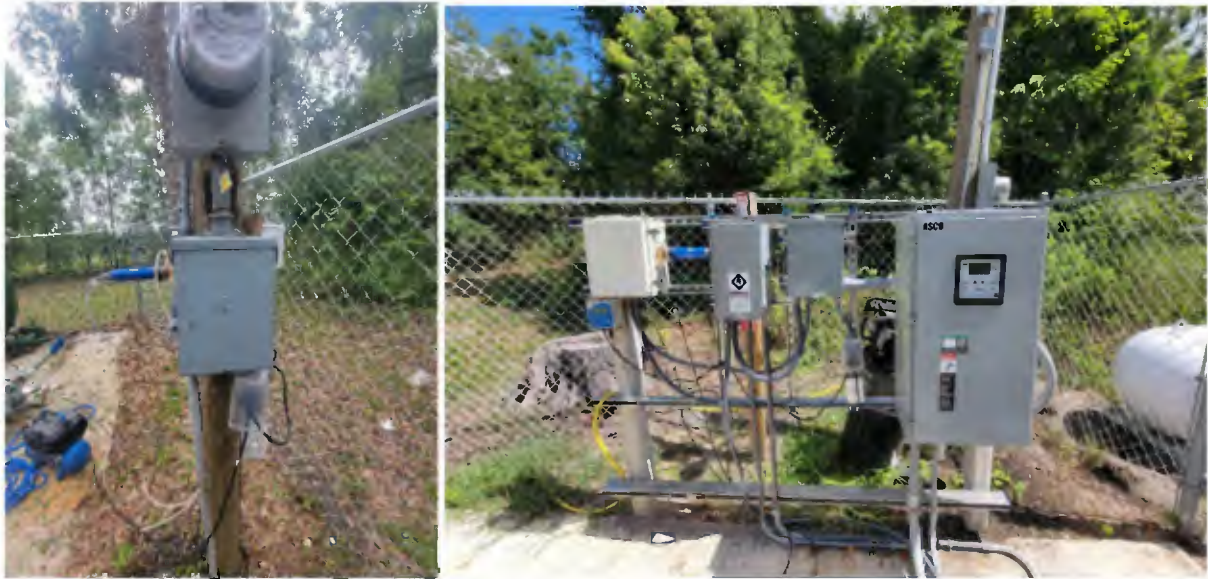
Before (Left) & After (Right): Electrical Panel Improvements - Eleven Oaks system.
