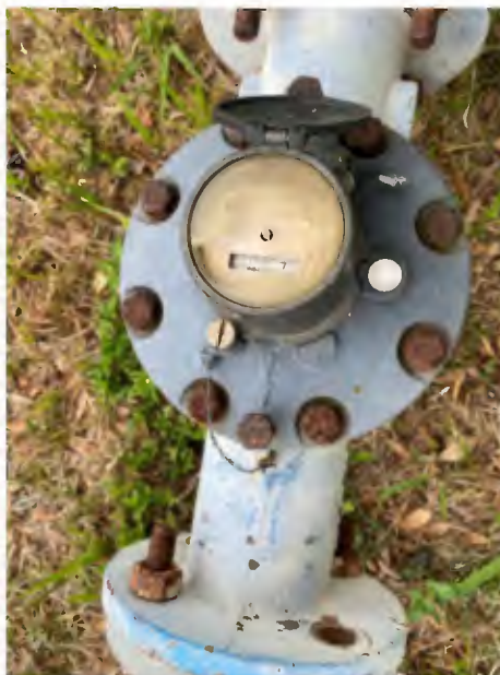
Figure 2-5: Broken Distribution Meter
