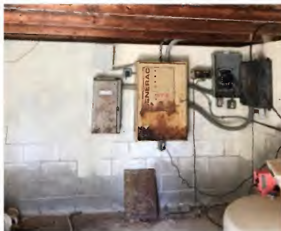
Figure 2-10: Automatic Transfer Switch
