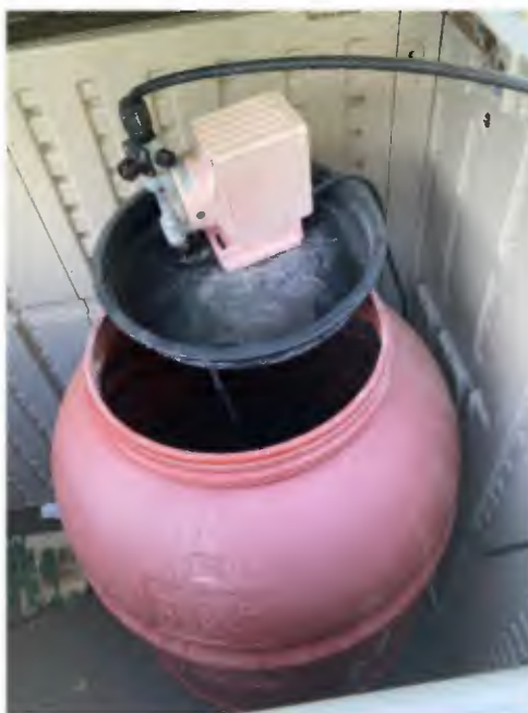
Figure 2-2: Chlorine Treatment Tank
