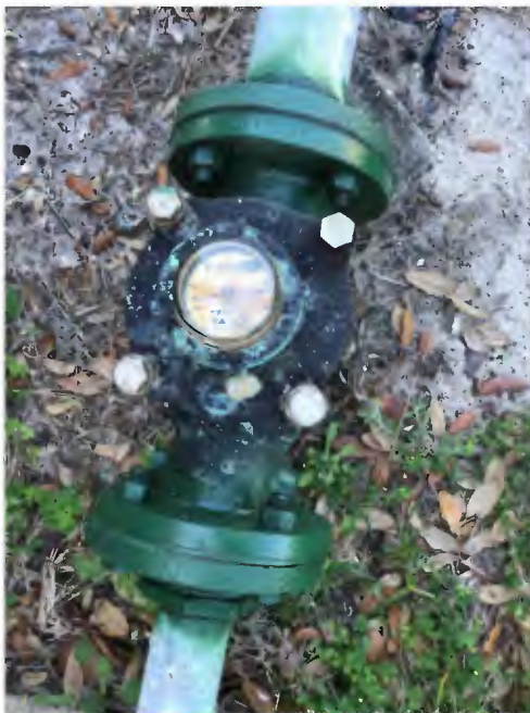
Figure 2-4: Terrace Well Source Meter
