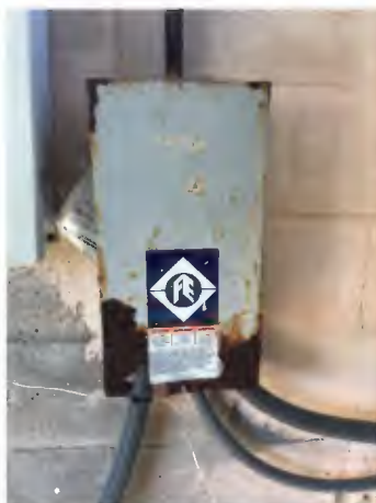
Figure 2-7: Rusted Well Starter Box
