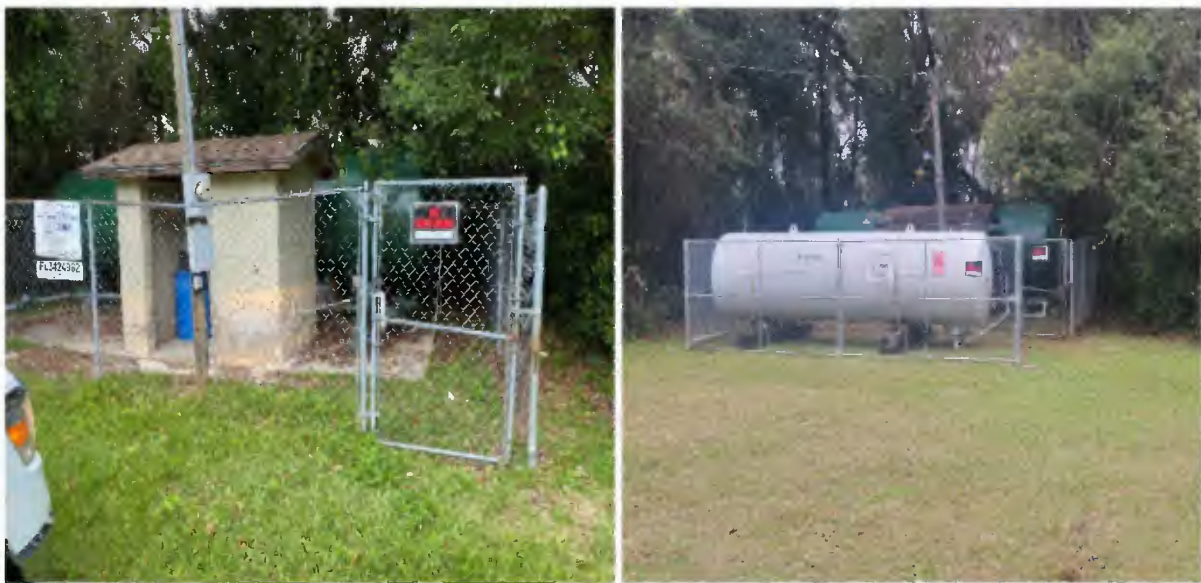
Before (Left) & After (Right): Hydro-pneumatic tank replacement (current tank leaking and at risk of failure) - Ashely Heights system.
