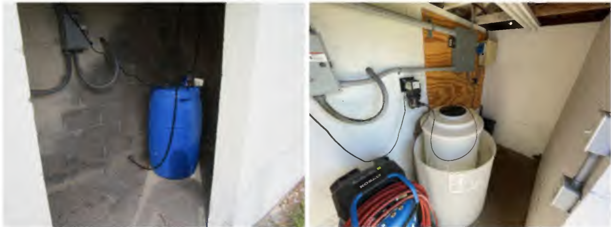
Before (Left) & After (Right): Disinfection improvements, containment and lighting - Country Walk system.
