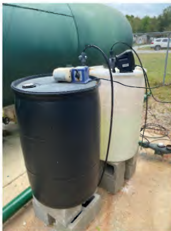
Figure 2-3: Chlorine Treatment
