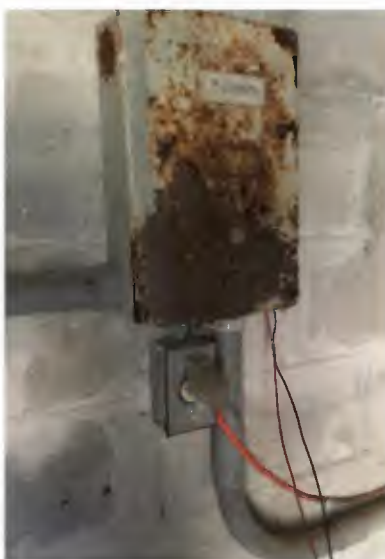
Figure 2-14: Pines WTP Well Pump Starter
