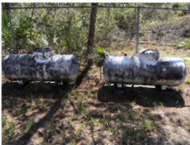
Figure 2-11: Propane Storage Tanks
