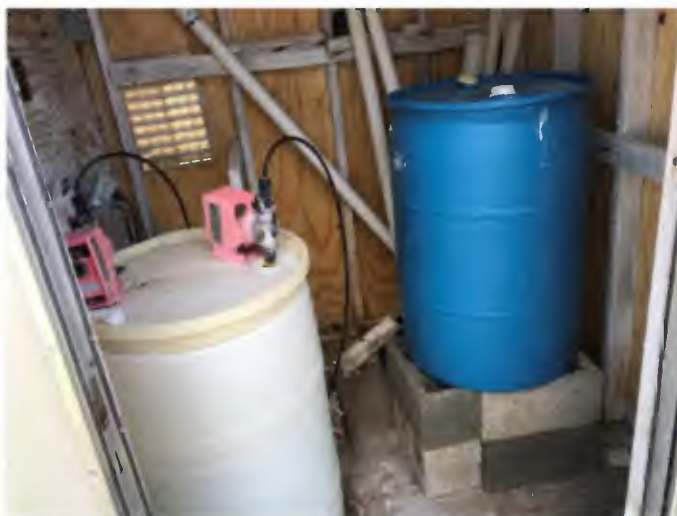
Figure 2-4: Chemical Pump Outlet
