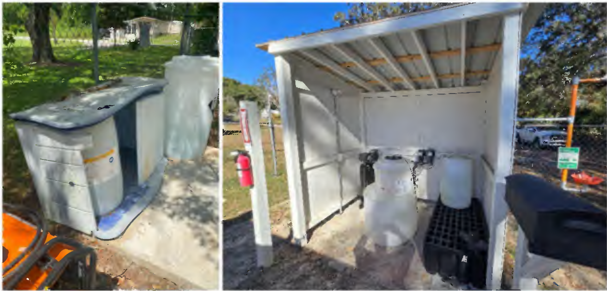
Before (Left) & After (Right): New Chemical containment and shade structure - Ponderosa Pines system.
