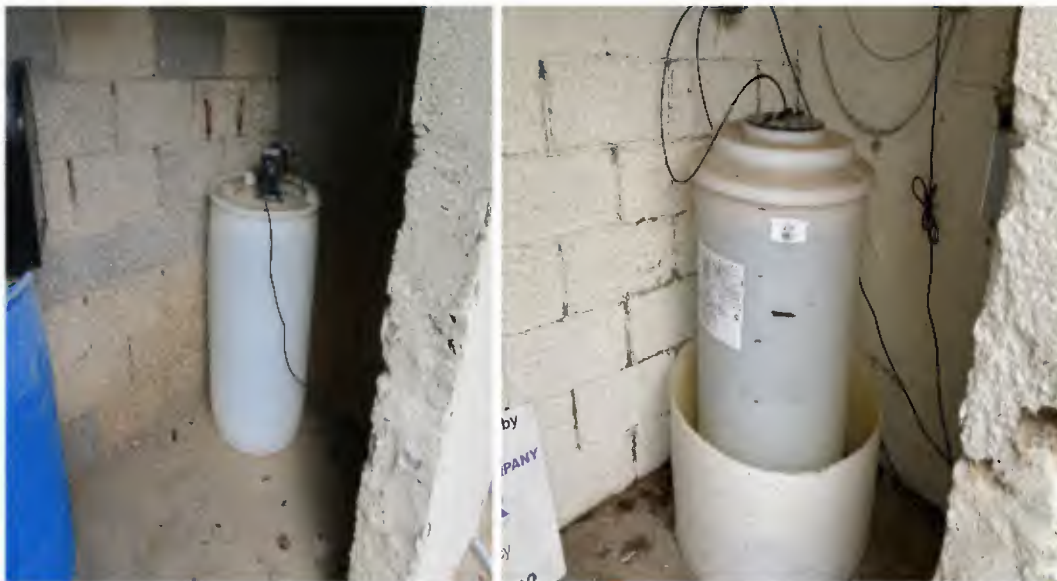
Before (Left) & After (Right): Chemical containment upgrades - Asheley Heights system.
