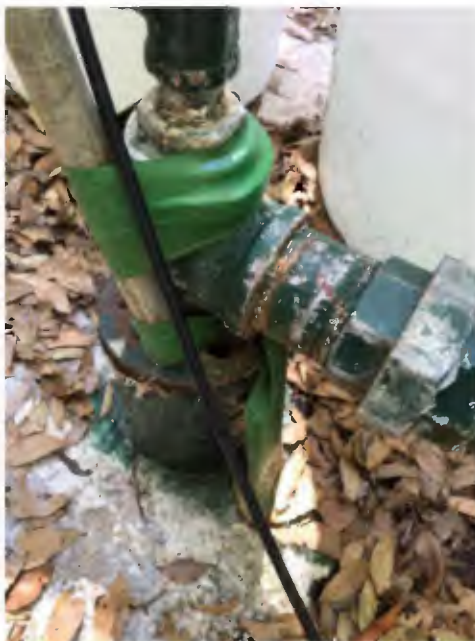
Figure 2-7: Unsealed Wellhead
