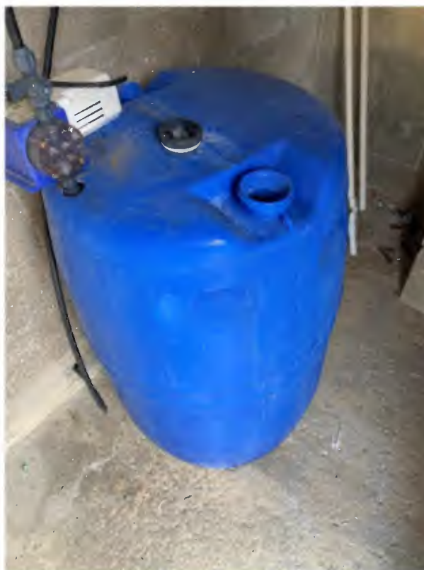
Figure 2-3: Chlorine Treatment
