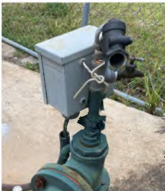
Figure 2-8: Well 2 Exposed Conduit Wire and Unscreened Vent
