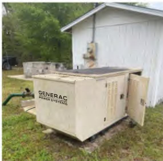
Figure 2-8: Back-up Power Generator
