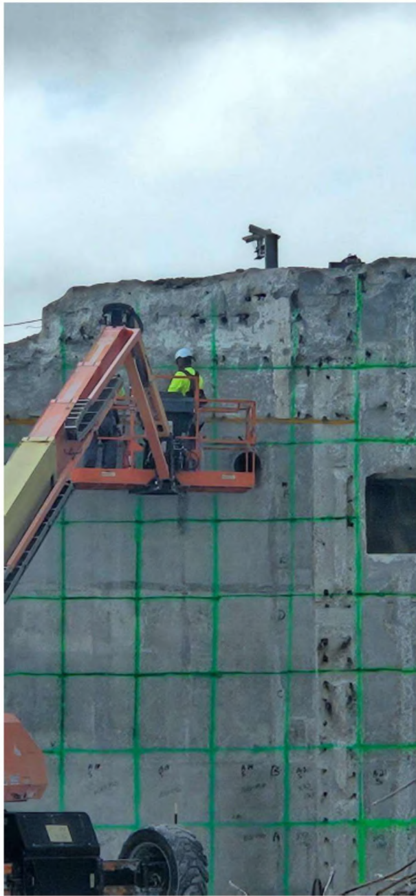
Scanning Auxiliary Building Wall
