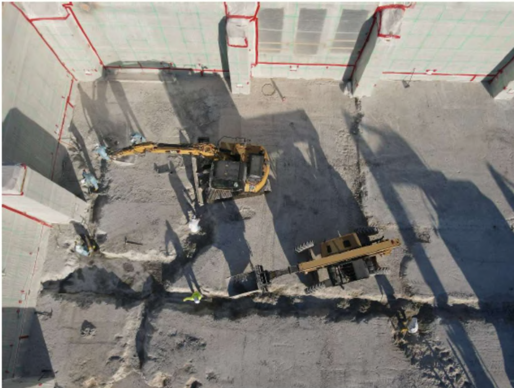
Turbine Building Drain Removal
