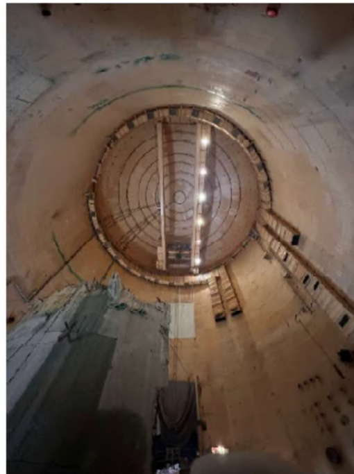
RB Spray Header Demolition
