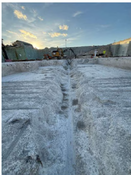
Auxiliary Building Substructures Drain Removal and Surveys
