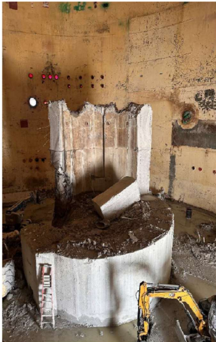
RB Bio-Shield Segmentation
