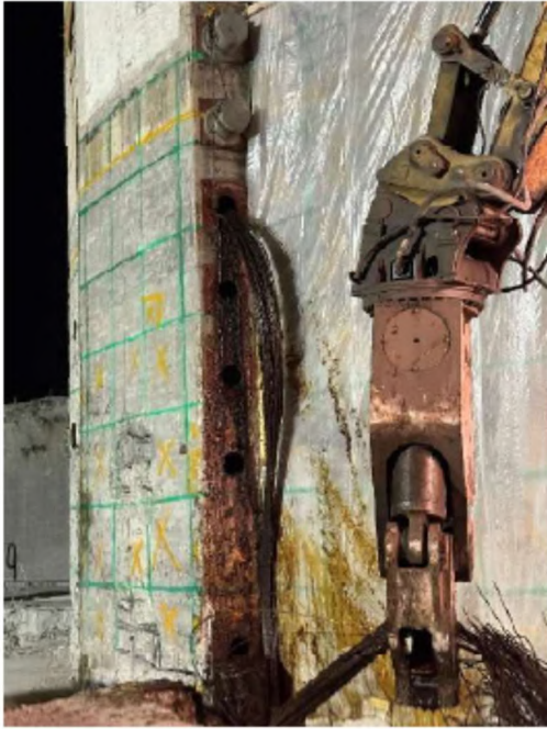
RB Horizontal Tendon Removal
