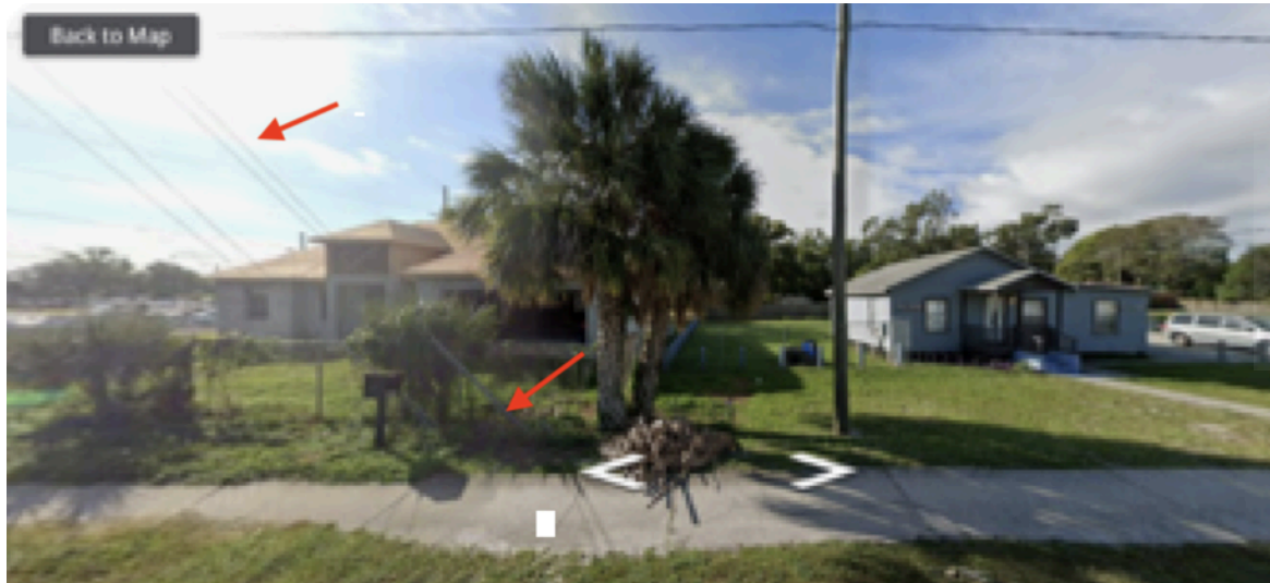
Before Photograph – Original Pole and Guy Wire Placement (Shows obstruction of garage access on adjacent property prior to driveway construction)
