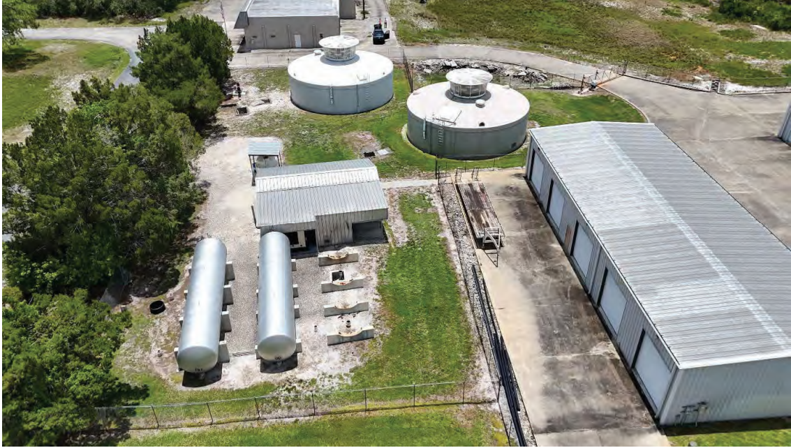
Photo #1 – Water Treatment Plant - Aerial View
