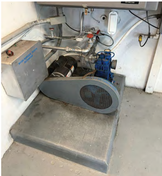
Photo # 52, 53 – Hydropneumatic Tanks Compressors (Outdoor)
