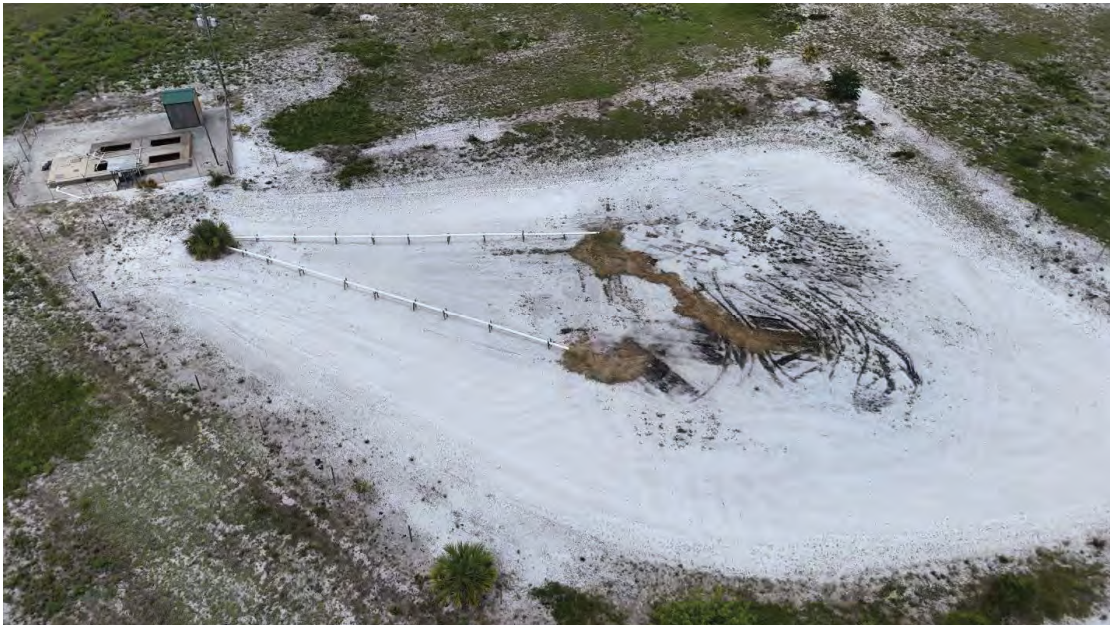
Photo # 61 – Rapid Infiltration Basin (RIB)
