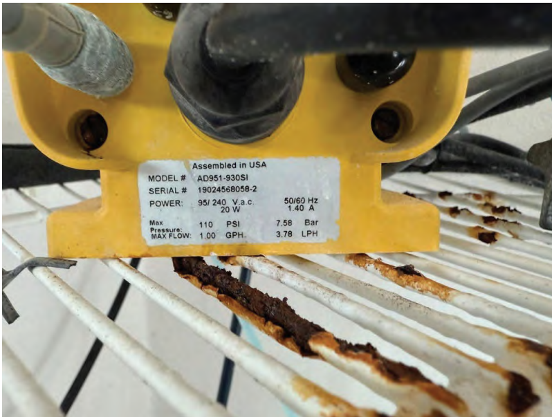
Photo # 39,40,41 – Corrosion Inhibitor System
