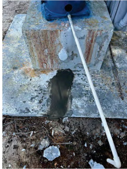
Photo 26: Well #1 Cracked Pad Repaired
