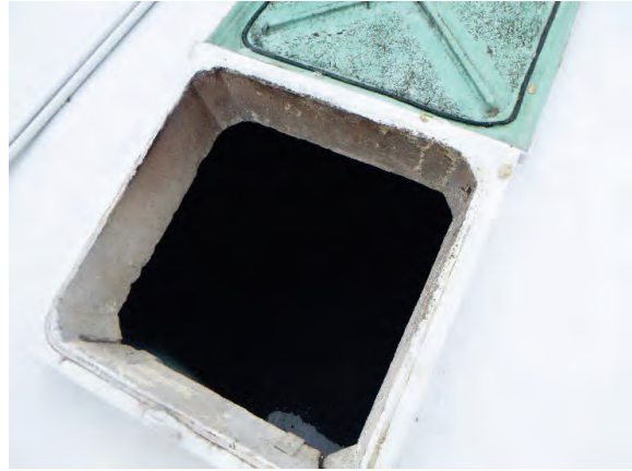
Photo 14: Ground Storage Tank #1 Manhole
