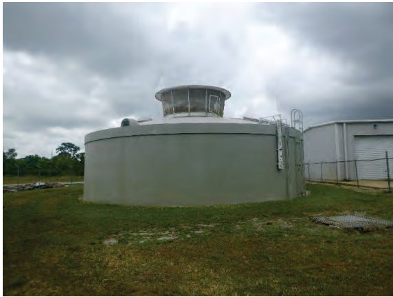
Photo 15: Ground Storage Tank #2
