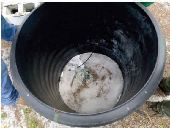
Photo 23: Corrosion Control Injection Site
