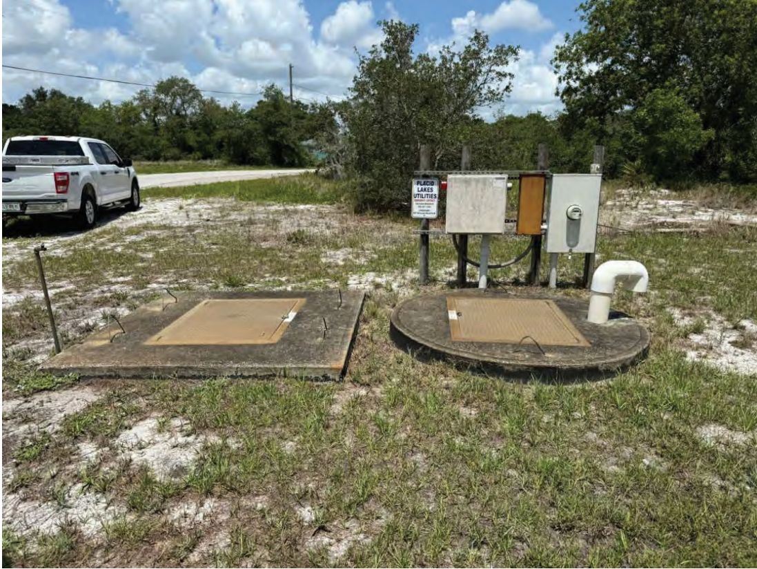
Photo # 71 – Lift Station No. 2 (Condos)
