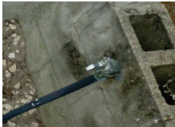
Photo 10: Well #3 Smooth-Nose Raw Water Sample Tap
