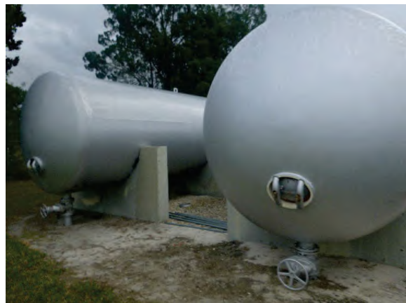
Photo 18: Hydro-Pneumatic Tanks #1 & #2
