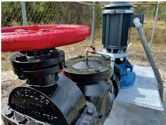
Photo 27: Well #2 Raw Water Tap Downward Facing
