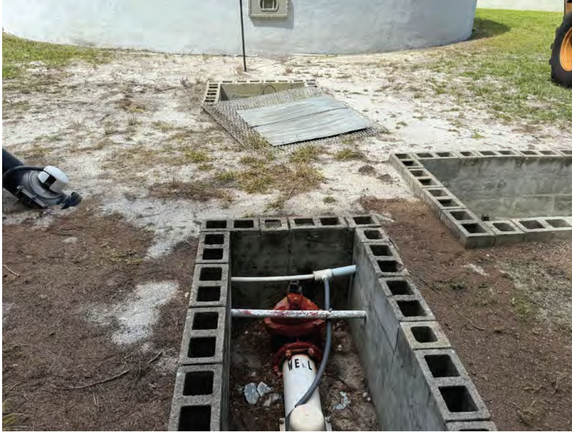
Photo #13 – Yard Vaults North-East of GSR No.1
