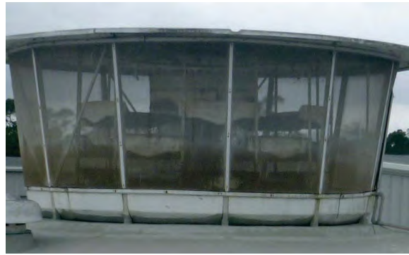
Photo 16: Ground Storage Tank #2 Aerator
