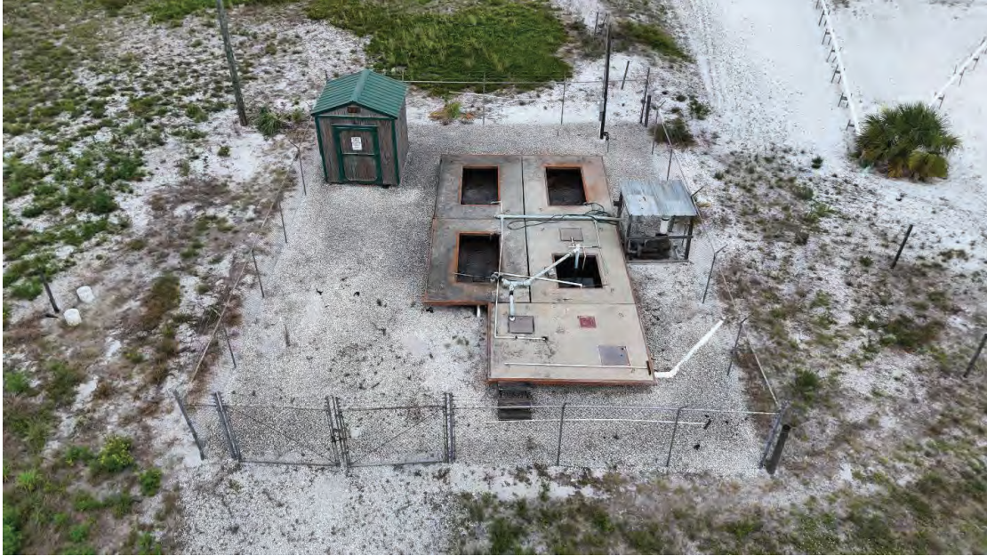
Photo # 60 – Wastewater Treatment Facility
