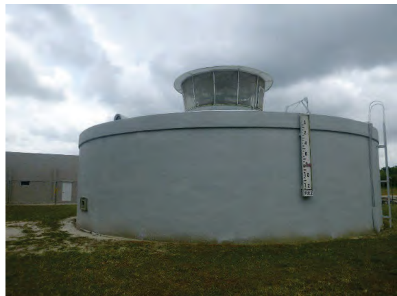
Photo 12: Ground Storage Tank #1
