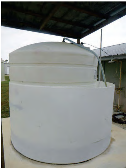
Photo 17: Chlorine Storage Container
