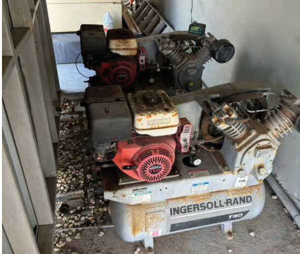
Photo # 52, 53 – Hydropneumatic Tanks Compressors (Outdoor)
