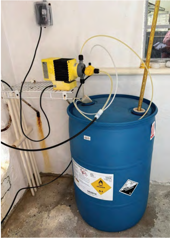
Photo # 42, 43 – Hydrogen Peroxide System
