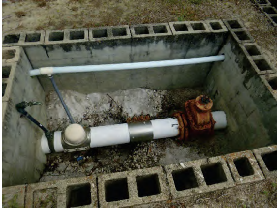
Photo 7: Well #2 Raw Water Sample Tap
