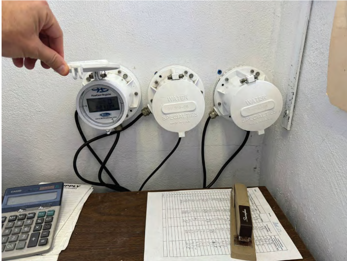
Photo # 38 – Wells Flowmeter Display
