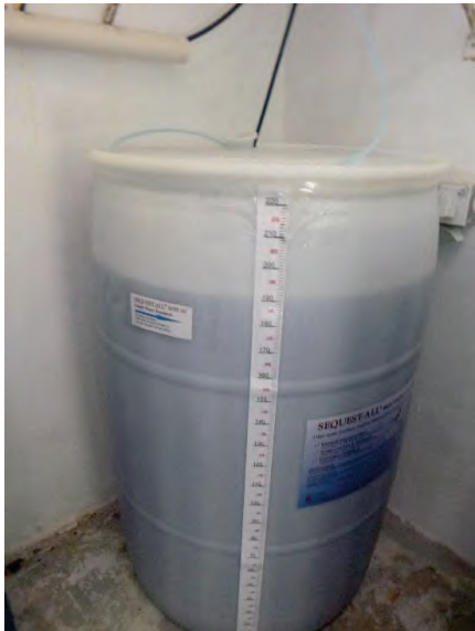
Photo 21: Sequest-All Corrosion Control Storage
