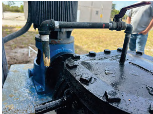
Photo 28: Well #1 Raw Water Tap Downward Facing
