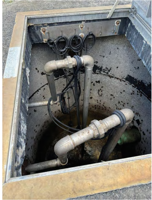
Photo # 75,76 – Lift Station No. 2 Wetwell (Condos) Valve Vault and Wetwell
