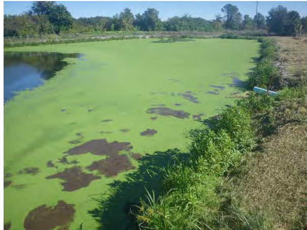
2 Sludge in percolation pond
