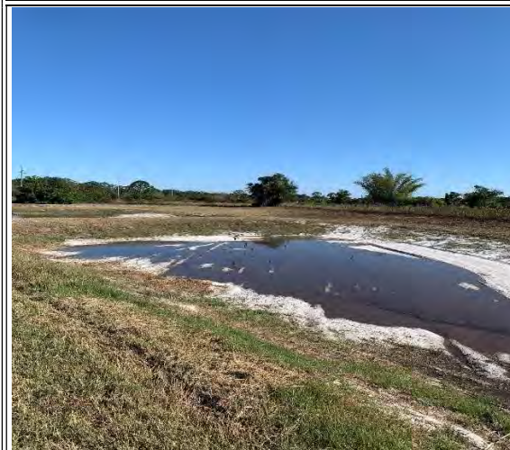
27. Rapid Infiltration Basin
