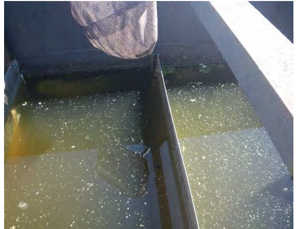
16 Separated baffle in CCC
