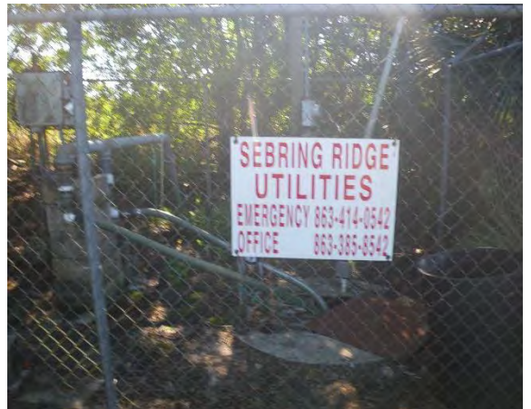
18 Clam Dr. lift station sign
