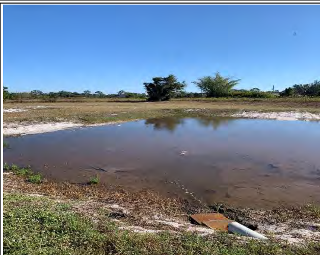
28. Rapid Infiltration Basin
