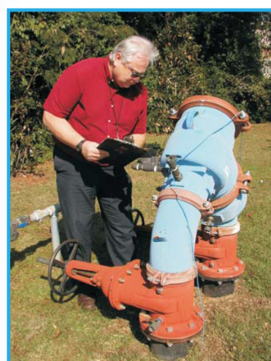
PSC engineer in the field
