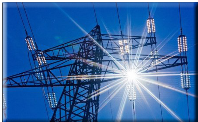
The 2019 Florida Legislature passed SB 796 to enact Section 366.96, F.S., entitled “Storm protection plan cost recovery.”
