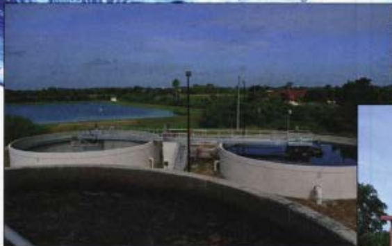
These clarifier tanks (above) and reuse water chlorine contact chambers (right) are part of the water and wastewater facilities at MacDill Air Force Base near Tampa, Fla. Ownership and maintenance of the facilities were transferred to the Florida Governmental Utility Authority, a "hybrid" governmental unit that will supply water and sewer services to approximately 20,000 people.
