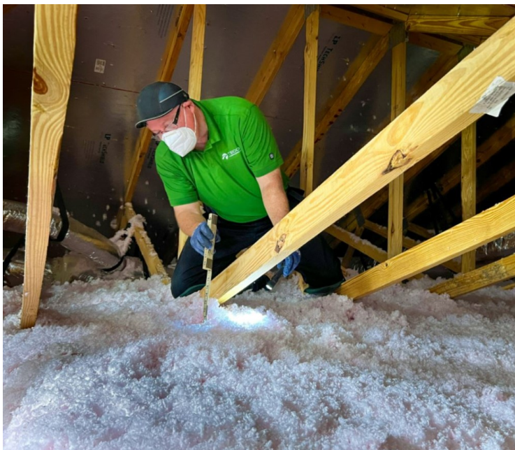
(Tampa Electric Residential Energy Analyst taking ceiling insulation depth measurements)
