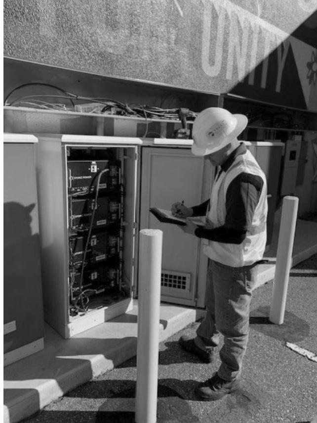
Commercial Energy Analyst inspecting BESS at McDonald Training Center
