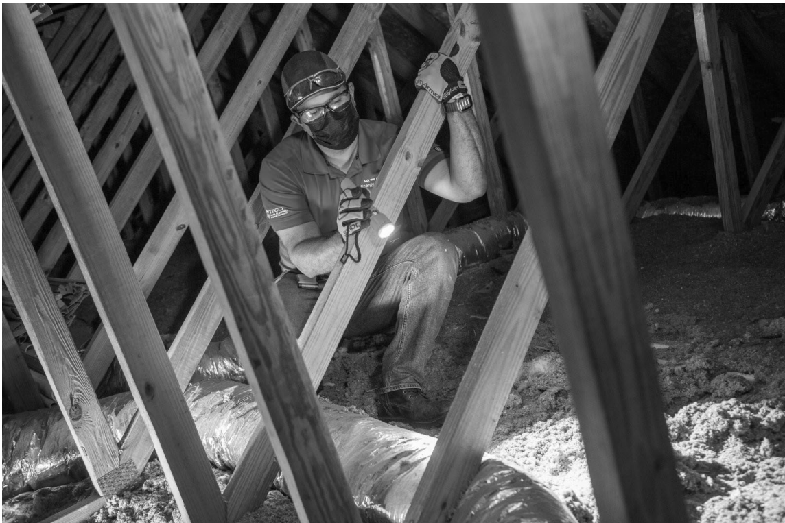
Residential Energy Analyst inspecting duct work in a customer attic.
