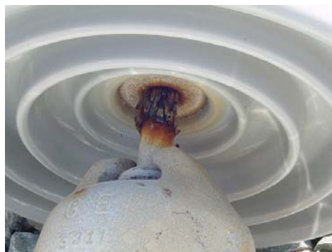
Typical State 4 “Ball & Socket” Insulators
