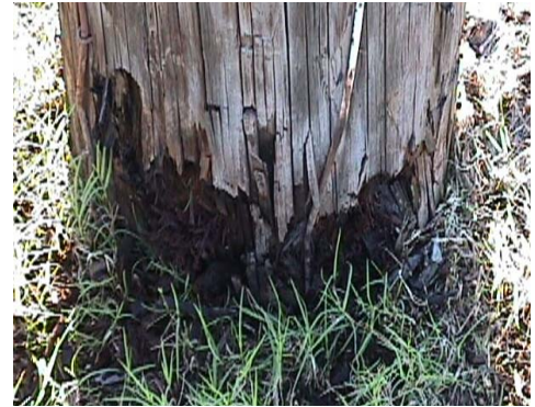
State 5 Groundline Pole Decay
