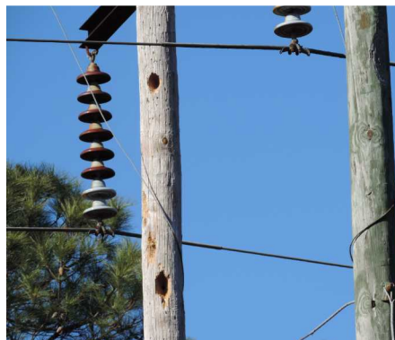
Priority 3 Woodpecker Holes (Not in critical locations)
