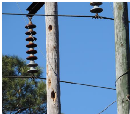
Priority 9 Woodpecker Holes (Not in critical locations)
