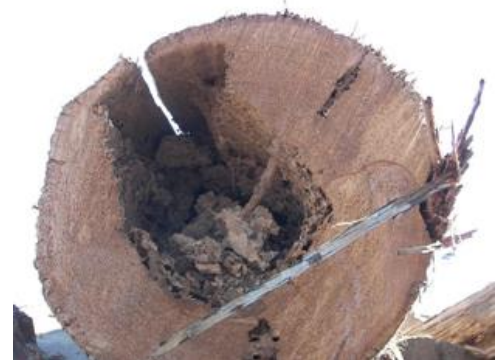
Priority 1 Internal Decay (Deep decay pocket)
