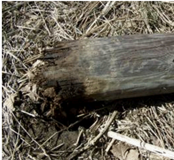
Green Growth (May be an indicator of substantial pole decay)
