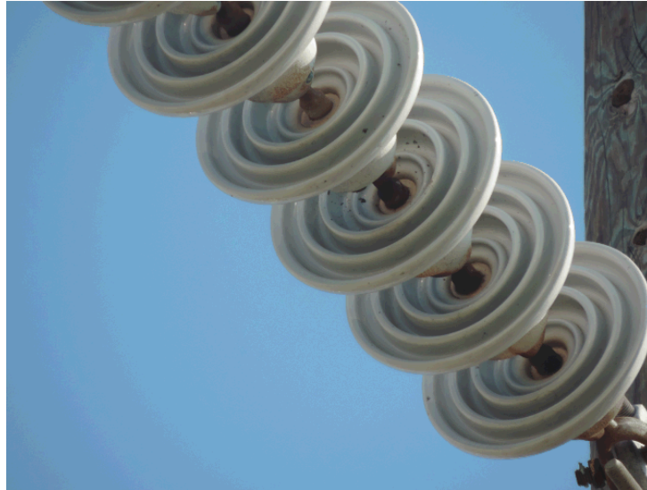
Priority 1 Porcelain Spark Erosion These can be difficult to see/evaluate
