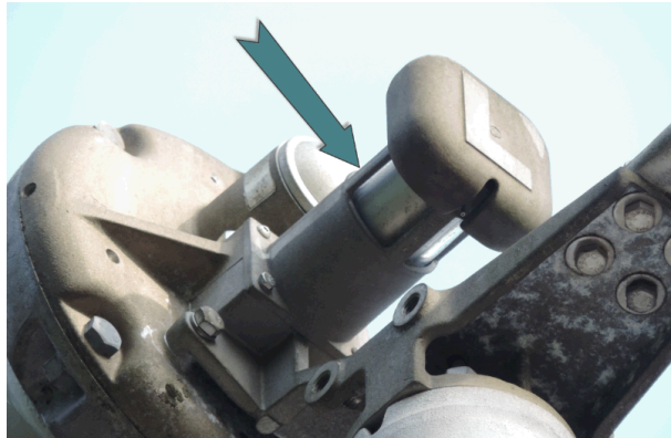
S&C Target is Normally White. Red Target Indicates Low Gas
