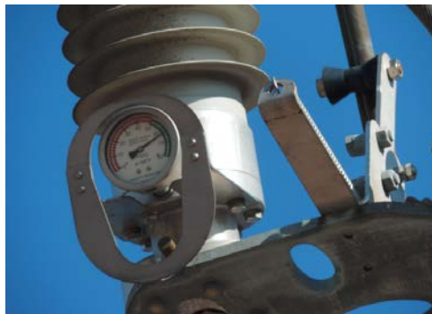
SF6 Gas Level on Southern States must be in the Green Region
