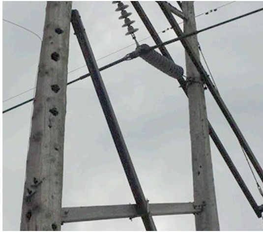
Priority 1 Woodpecker holes with large internal cavities
