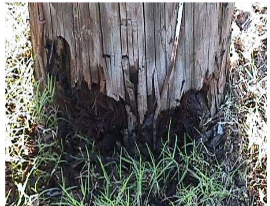
Priority 1 Groundline Pole Decay
