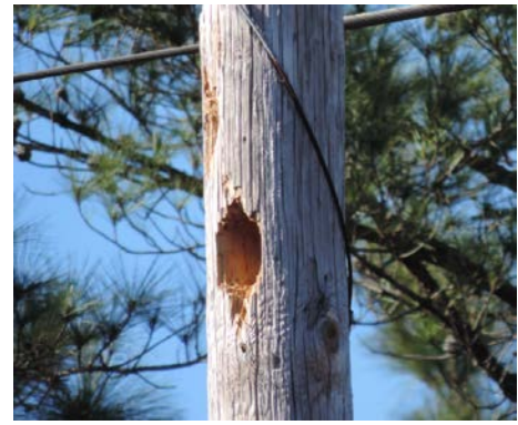
Priority 9 Woodpecker Hole (Does not hold water & can be repaired)
