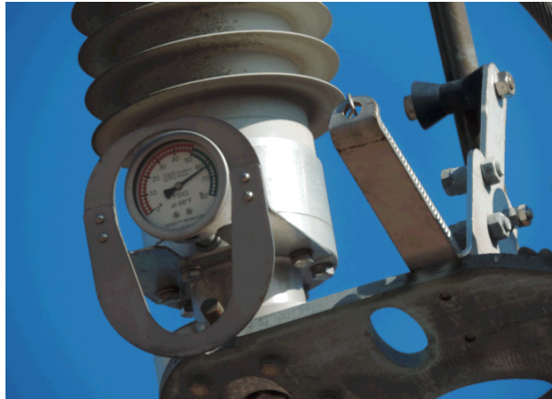
SF6 Gas Level on Southern States must be in the Green Region
