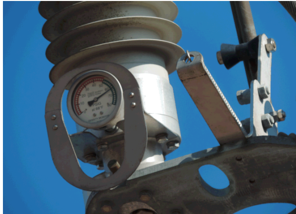
SF6 Gas Level on Southern States must be in the Green Region
