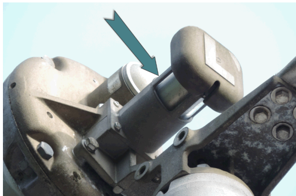
S&C Target is Normally White. Red Target Indicates Low Gas
