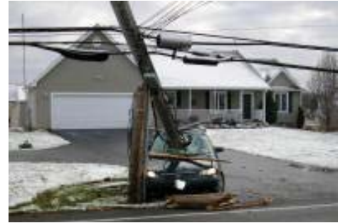
Motor vehicle versus utility pole may be dangerous
