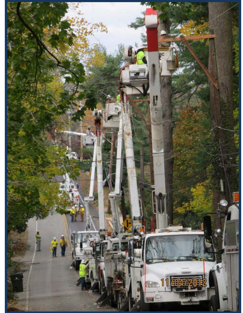
Line Crews in Pennsylvania
