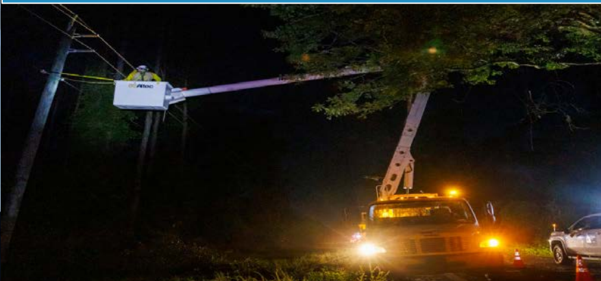
Night Work Overnight execution efficiency
