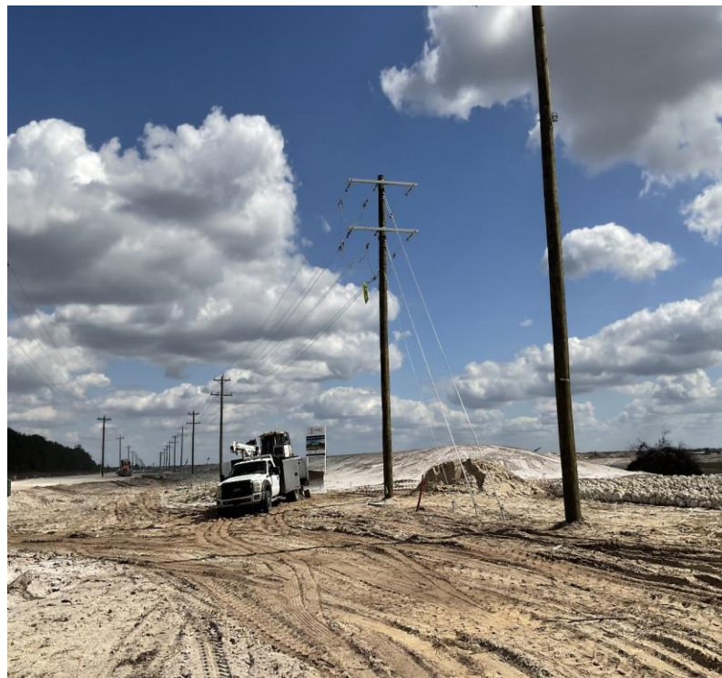
LCEC: New line infrastructure installed
