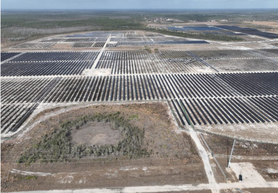
FIGURE 3.2 Bay Ranch Solar Power Plant
