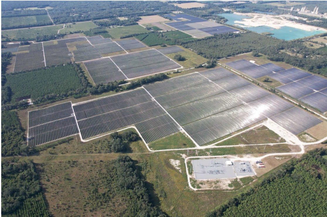
FIGURE 3.5 Hildreth Power Plant
