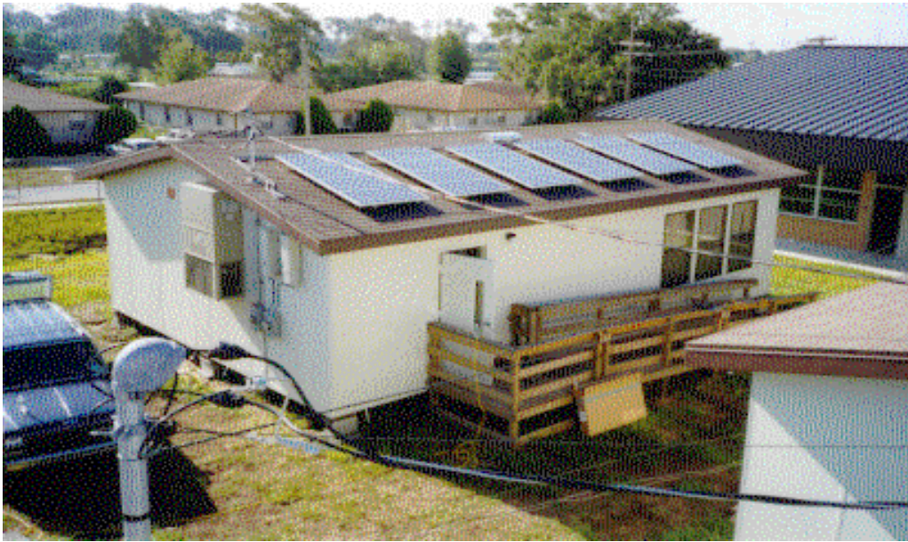
Figure 4-2 Portable Classroom Topped by PV Panels
