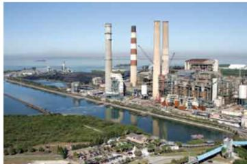
The station operates four (4) pulverized coal-fired steam units equipped with desulfurization scrubbers, electrostatic precipitators, and selective catalytic reduction (SCR) air pollution control systems. In addition, the station operates one (1) aero-derivative combustion turbine that entered into service in 2009 and can be fired with natural gas or distillate oil.
