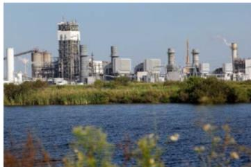
The station operates five (5) generating units. Polk Unit 1 is an integrated gasification combined cycle (IGCC) unit fired with synthetic gas produced from gasified coal and other carbonaceous fuels. This technology integrates state-of-the-art environmental processes to create a clean fuel gas from a variety of feedstock with the efficiency benefits of combined cycle generation equipment. Polk Units 2 through 5 are combustion turbines fired
