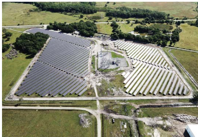
FIGURE 3.2 Osceola Solar Site
