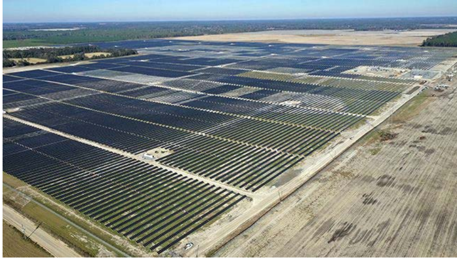
FIGURE 3.5 Hamilton Solar Site
