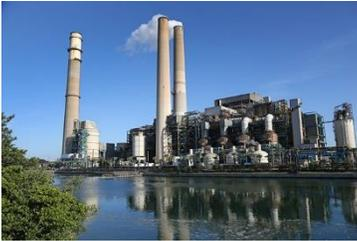
Big Bend Units 1-4 are four (4) pulverized coal-fired steam units equipped with desulfurization scrubbers, electrostatic precipitators, and Selective Catalytic Reduction (SCR) air pollution control systems. All four units can also be fired with natural gas. Big Bend CT 4 is one (1) aero-derivative combustion turbine that can be fired with natural gas or distillate oil.
