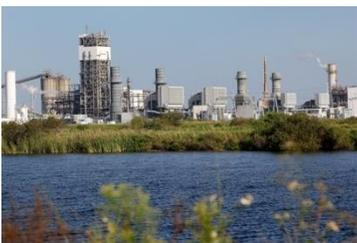
The station operates one (1) integrated coal gasification combined cycle (IGCC) unit and one (1) natural gas-fired combined cycle unit. Polk Unit 1 is an IGCC unit fired with synthetic gas produced from gasified coal and other carbonaceous fuels. This technology integrates state-of-the-art environmental processes to create a clean fuel gas from a variety of feedstock with the efficiency benefits of combined cycle generation equipment. Unit 1 can also be fired with natural gas. Polk 2 Combined
