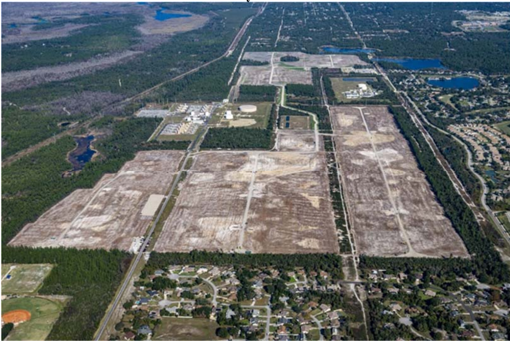
FIGURE 3.8 DeBary Solar Site
