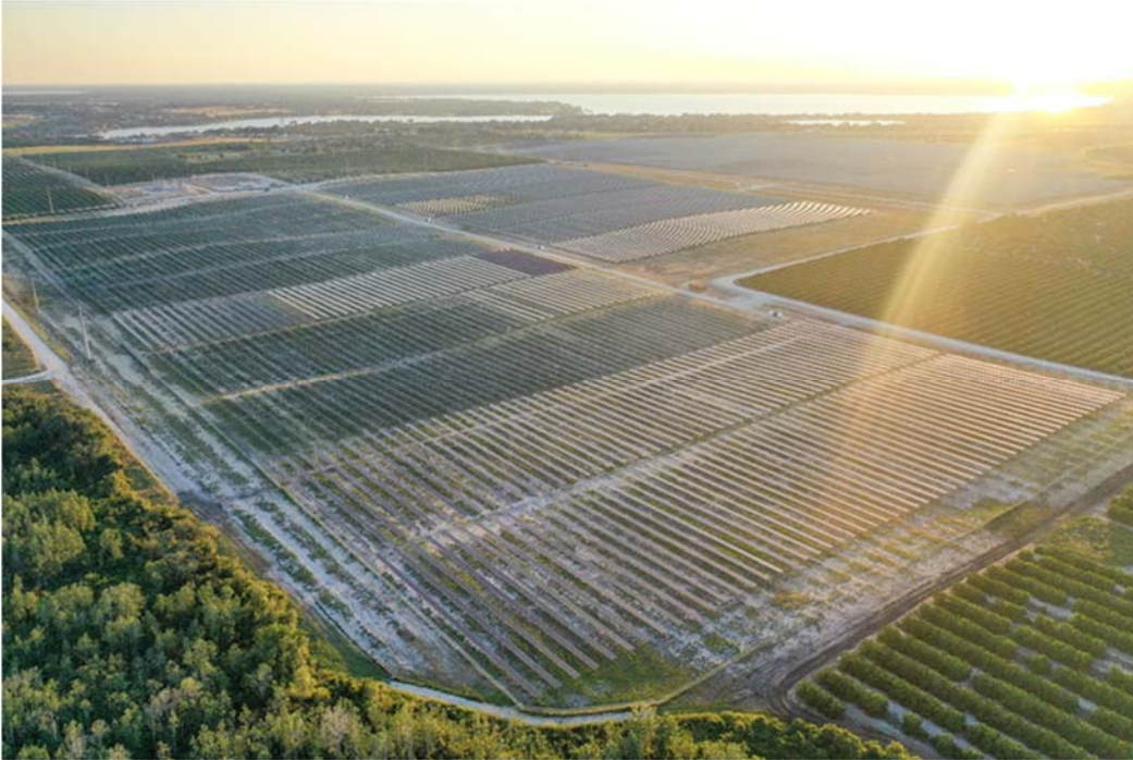
FIGURE 3.6 Lake Placid Solar Site
