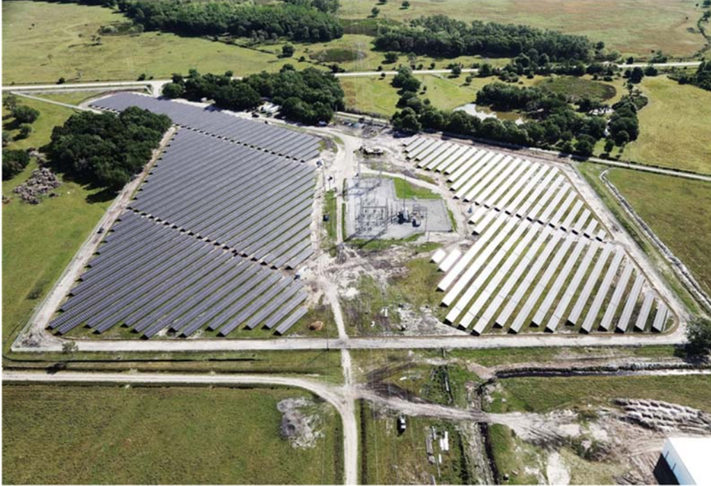
FIGURE 3.2 Osceola Solar Site
