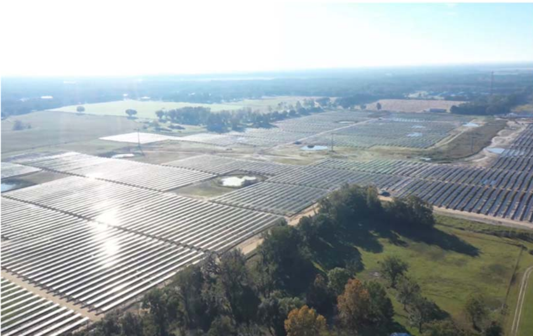
FIGURE 3.7 Trenton Solar Site
