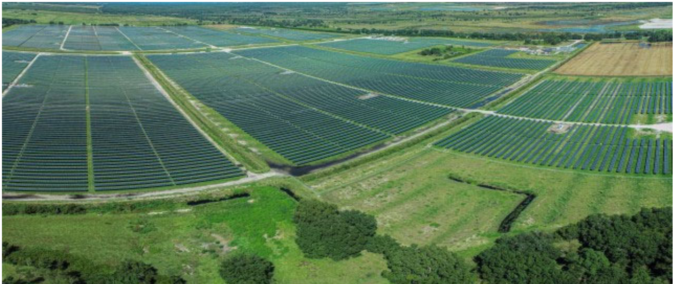
FIGURE 3.4 Duette Solar Power Plant
