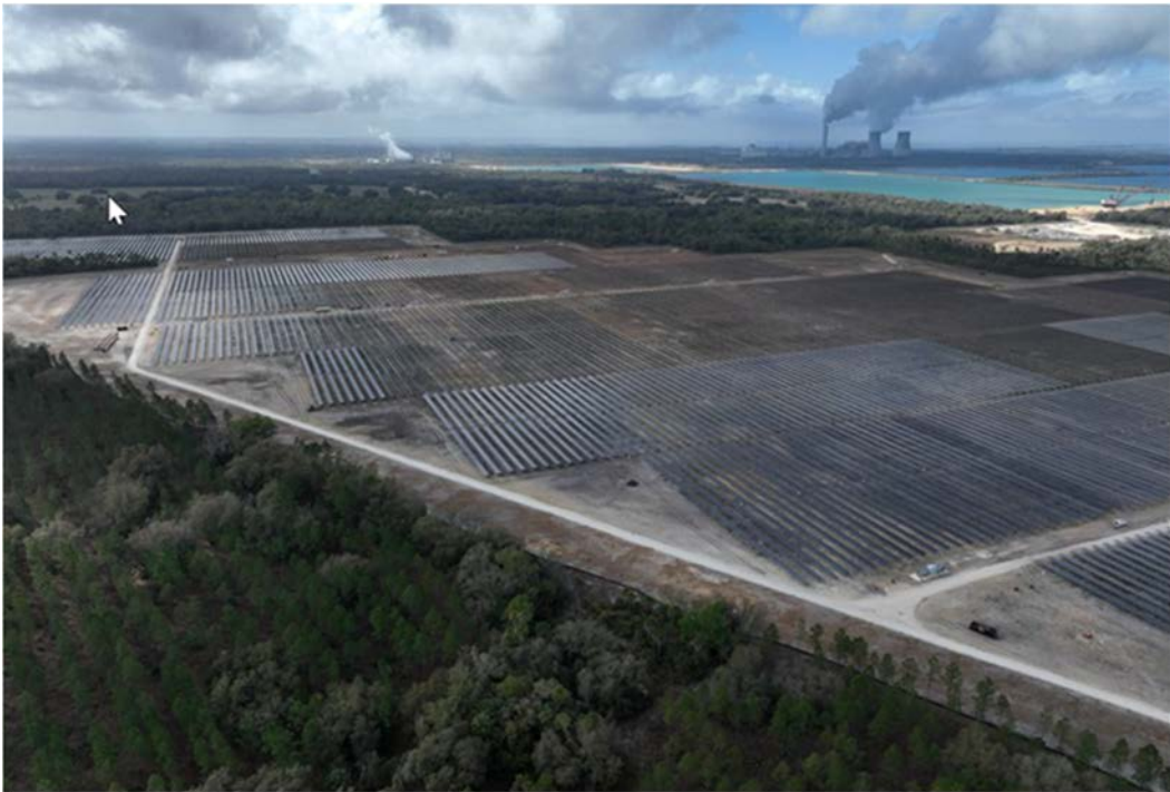
FIGURE 3.5 Bay Trail Solar Power Plant
