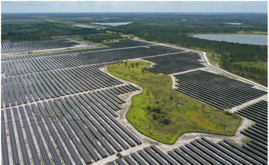
FIGURE 3.3 Fort Green Solar Power Plant
