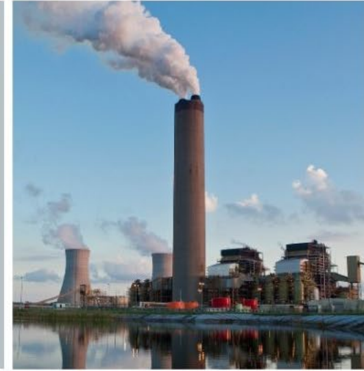
Midulla Generating Station (MGS) 949 MW natural gas facility.
